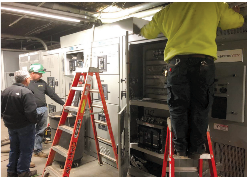
REPLACEMENT OF OIT'S SUB-BASEMENT ELECTRICAL GEAR AND TRANSFORMER THAT SUPPORTS ELECTRICAL POWER FOR OIT'S DATA CENTER, THE CENTRAL HUB OF THE CITY'S NETWORK AND MISSION CRITICAL APPLICATIONS.
