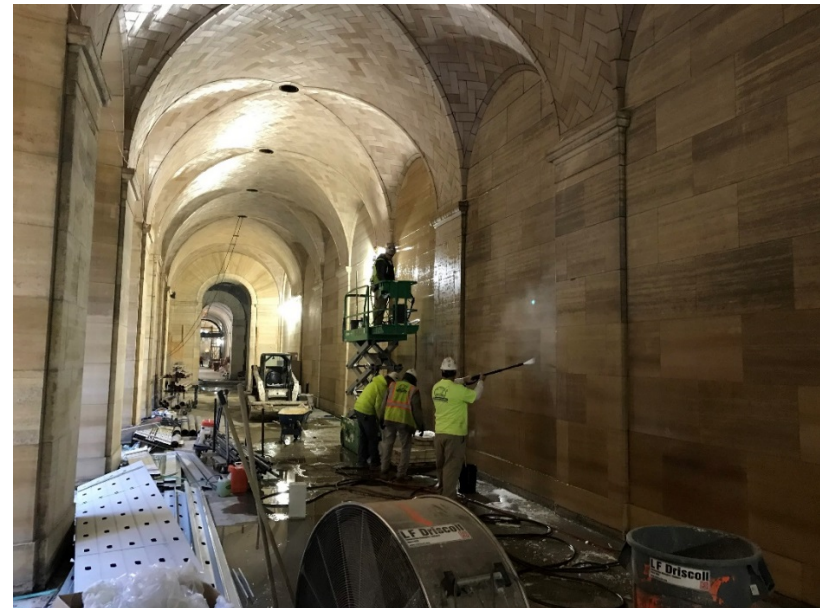
The long-closed Vaulted Walkway on Level C is currently undergoing restoration as part of the Core Project.
