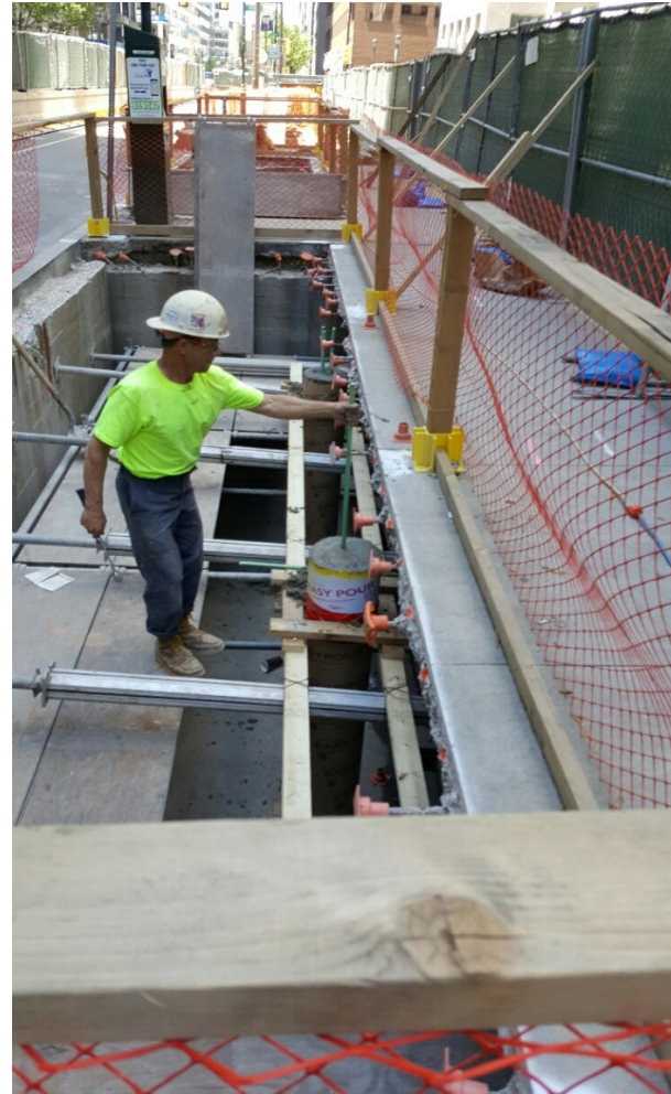
DPP-managed restoration of underground vent structures and sidewalk grates along Market Street, Center City
