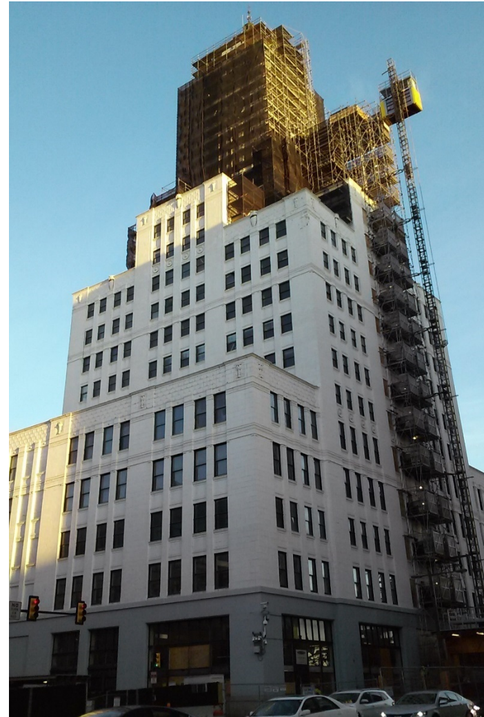
Exterior work underway on the transformation of 400 North Broad Street into the Philadelphia Public Safety Building.
