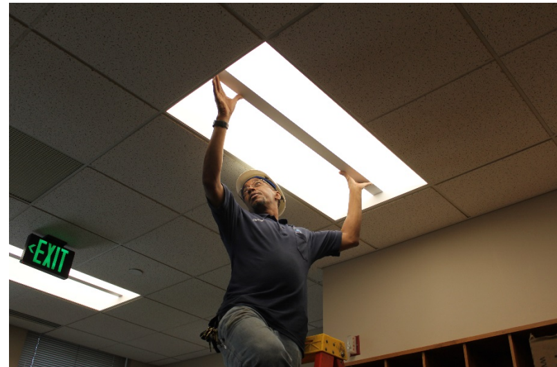
Installation of LED lighting in the One Parkway Building
