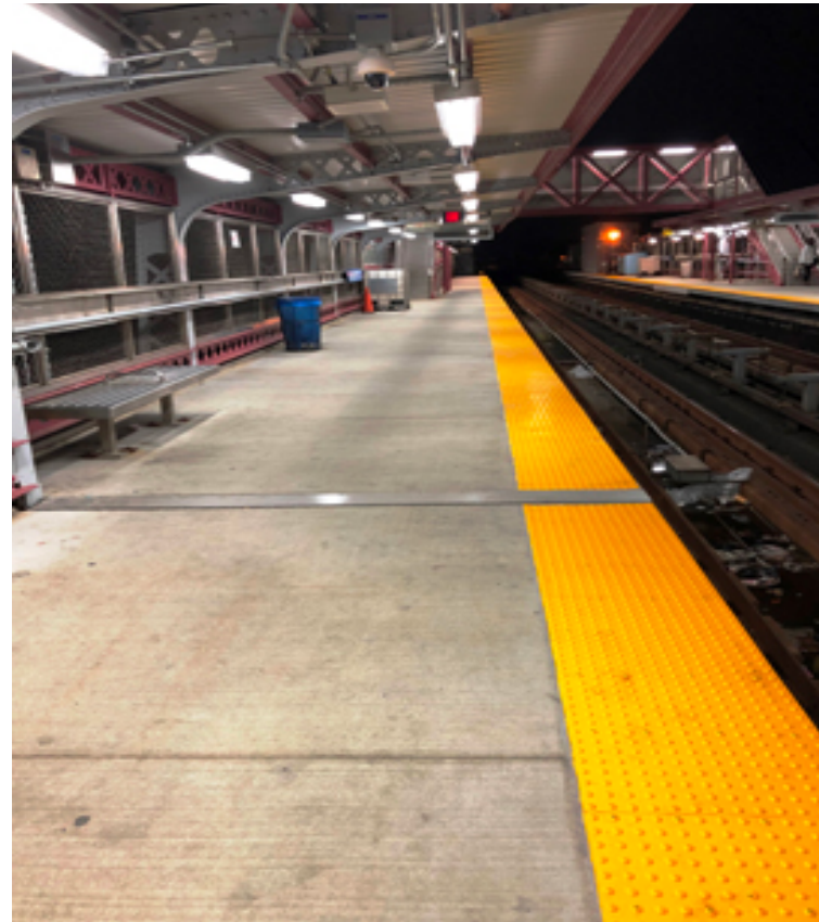
Rehabilitated canopy, roof, lighting, and platform at the Market-Frankford Line's Arrott Transportation Center in Frankford.
