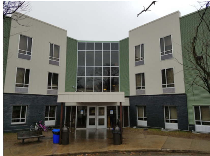
Recent exterior improvements to the Woodstock Family Center, North Philadelphia
