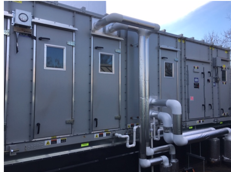
New air handling equipment at the PECO Primate Reserve, Philadelphia Zoo, West Philadelphia
