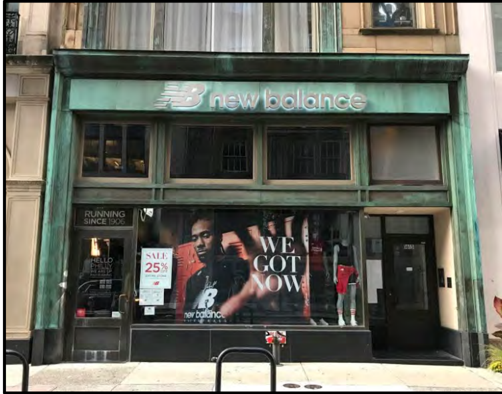
Figure 48. The Primary (South) Elevation of the subject property, showing the first-floor storefront. Source: Tim Kerner, 2020.
