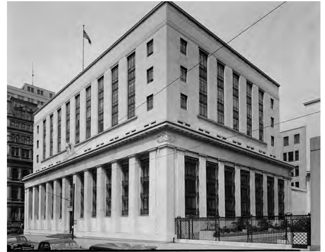
Image 8: Historic Photo showing existing Garden Court from Chestnut Street
