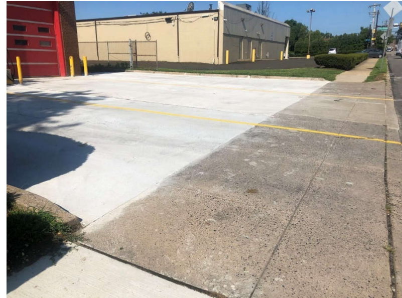
New concrete apron for Fire Department apparatus at Engine 58 on Hendrix Street, Somerton.
