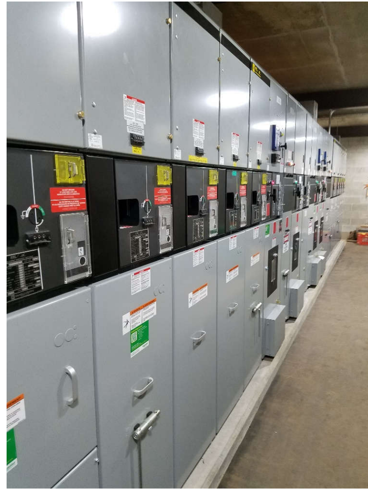
Newly installed electric switchgear for Department of Prisons facilities.
