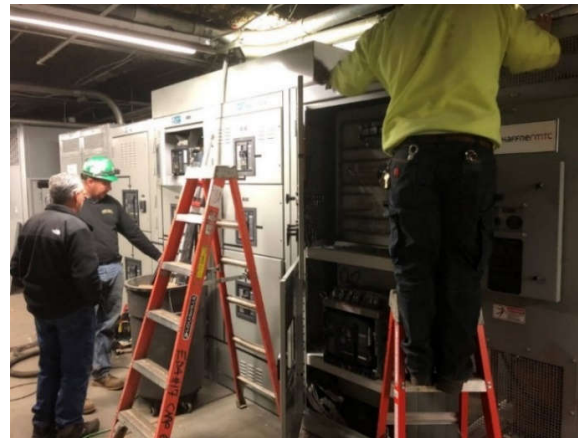
Transformer replacement at the City's data center.
