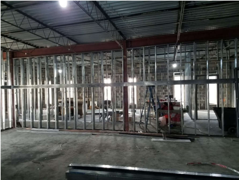
Interior framing underway for new Police District 2, Castor Avenue and Elgin Street, Northeast Philadelphia.
