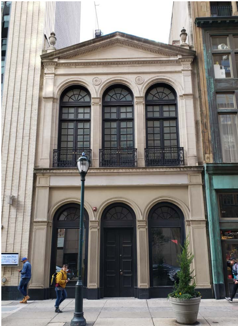
Figure 3. Walnut Street façade, 2019. (Source: Philadelphia Historical Commission)
