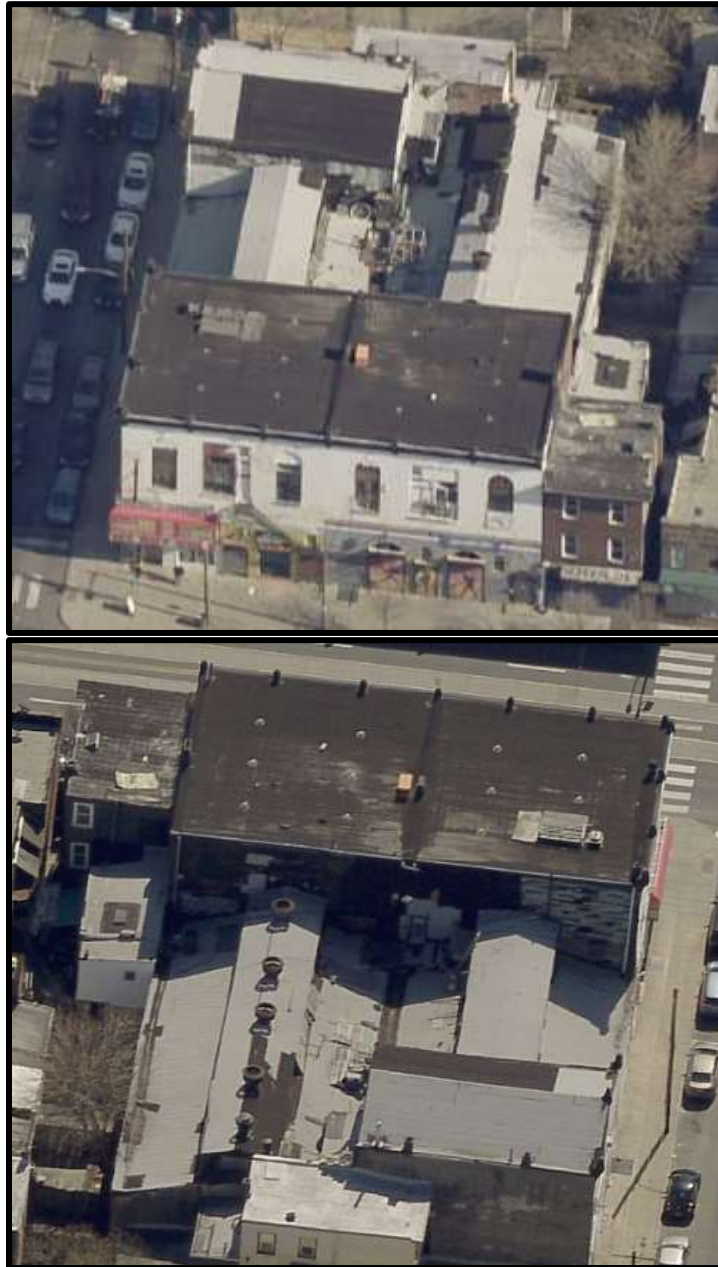
Figure 6. Top: Looking north at the primary (south) elevation. Figure 7. Bottom: Looking south at the market sheds of the subject property. Source: Pictometry, City of Philadelphia.
