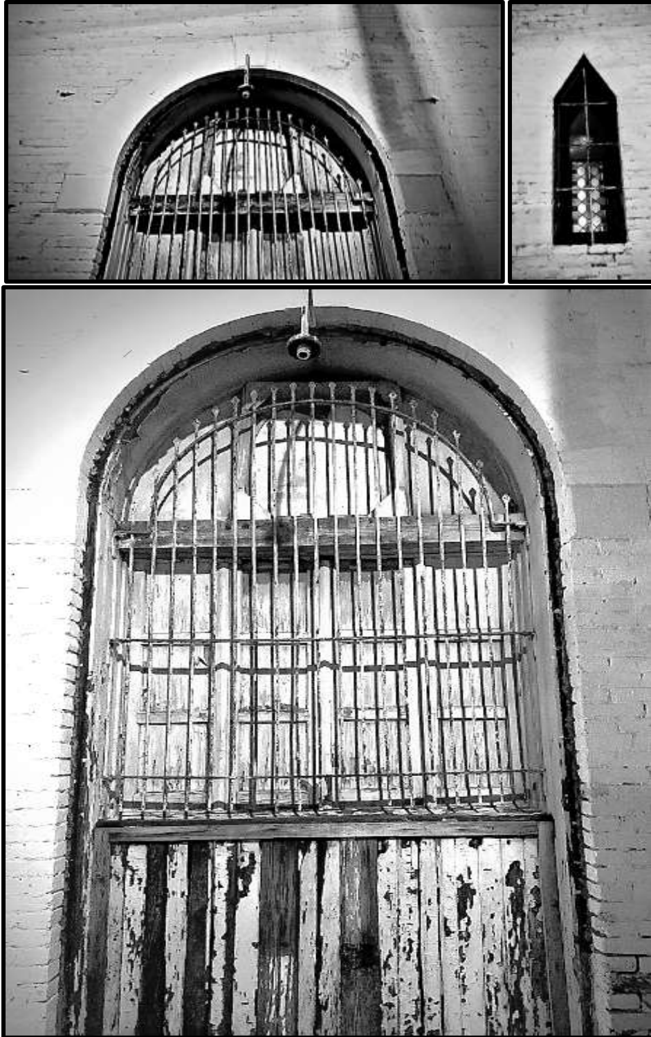
Figure 12. Top left: A representative brick arch with keystones and key blocks within the side (west) elevation. Figure 13. Top right: A window within the side (west) elevation featuring a triangular arch. Figure 14. Bottom: Original or early materials in one of the intact round arch doorways within the side (west) elevation. Source: Oscar Beisert, 2019.
