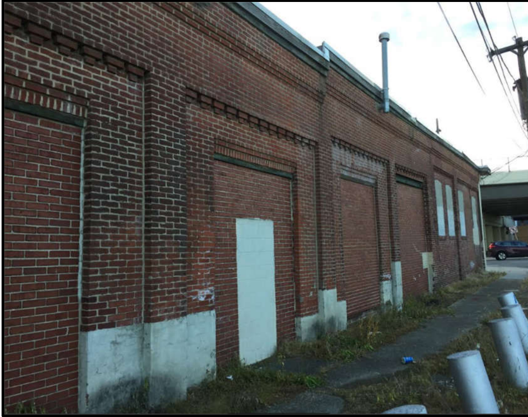
Figure 9. Bottom: the side (northeast) elevation. Source: Oscar Beisert, 2019.
