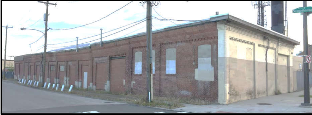
Figure 3. View from North Delaware Avenue at Susquehanna Avenue of the Empire Chain Works. Source: Oscar Beisert, 2019.
