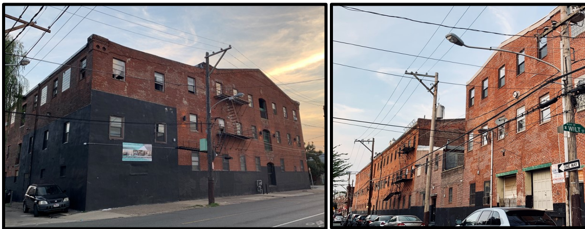
Figure 6. Left: The east and north elevations of Buildings 6a and 1. Figure 7. Right: The Howard Street Streetscape. Source: Oscar Beisert, 2019.
