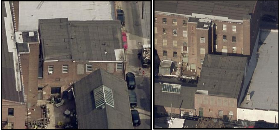
Figure 16. Left: Looking north at Buildings 3, 4, and 5. Source: Pictometry, Atlas, City of Philadelphia, 2018. Figure 17. Right: Looking west at Buildings 3, 4, and 5. Source: Oscar Beisert, 2019.
