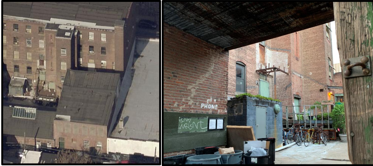
Figure 12. Left: Looking west at Buildings 3, 4, and 5. Source: Pictometry, Atlas, City of Philadelphia, 2018. Figure 13. Right: Looking into the court at the base of Building 2. Source: Oscar Beisert, 2019.
