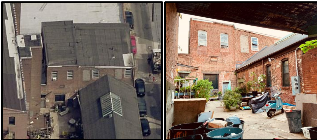
Figure 14. Left: Looking north at Buildings 3, 4, and 5. Source: Pictometry, Atlas, City of Philadelphia, 2018. Figure 15. Right: Looking into the court at Building 3 and 4. Source: Oscar Beisert, 2019.
