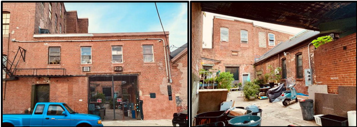
Figure 21. Left: Looking east Building 2. Figure 22. Right: Looking west at Building 2. Source: Pictometry, Atlas, City of Philadelphia, 2019.
