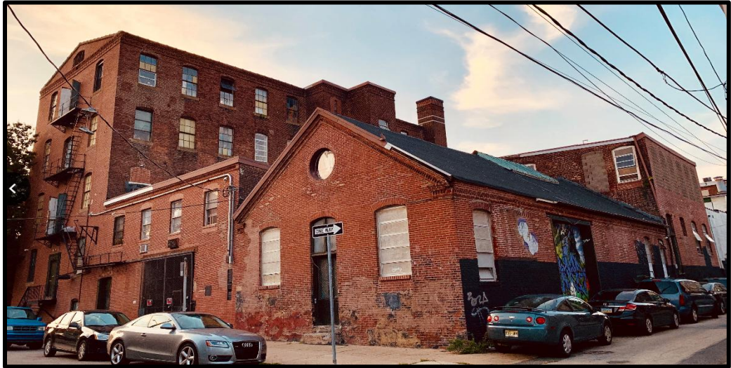
Figure 5. Looking northwest at the south and east elevations of the buildings and structures that comprise the subject property. Source: Oscar Beisert.
