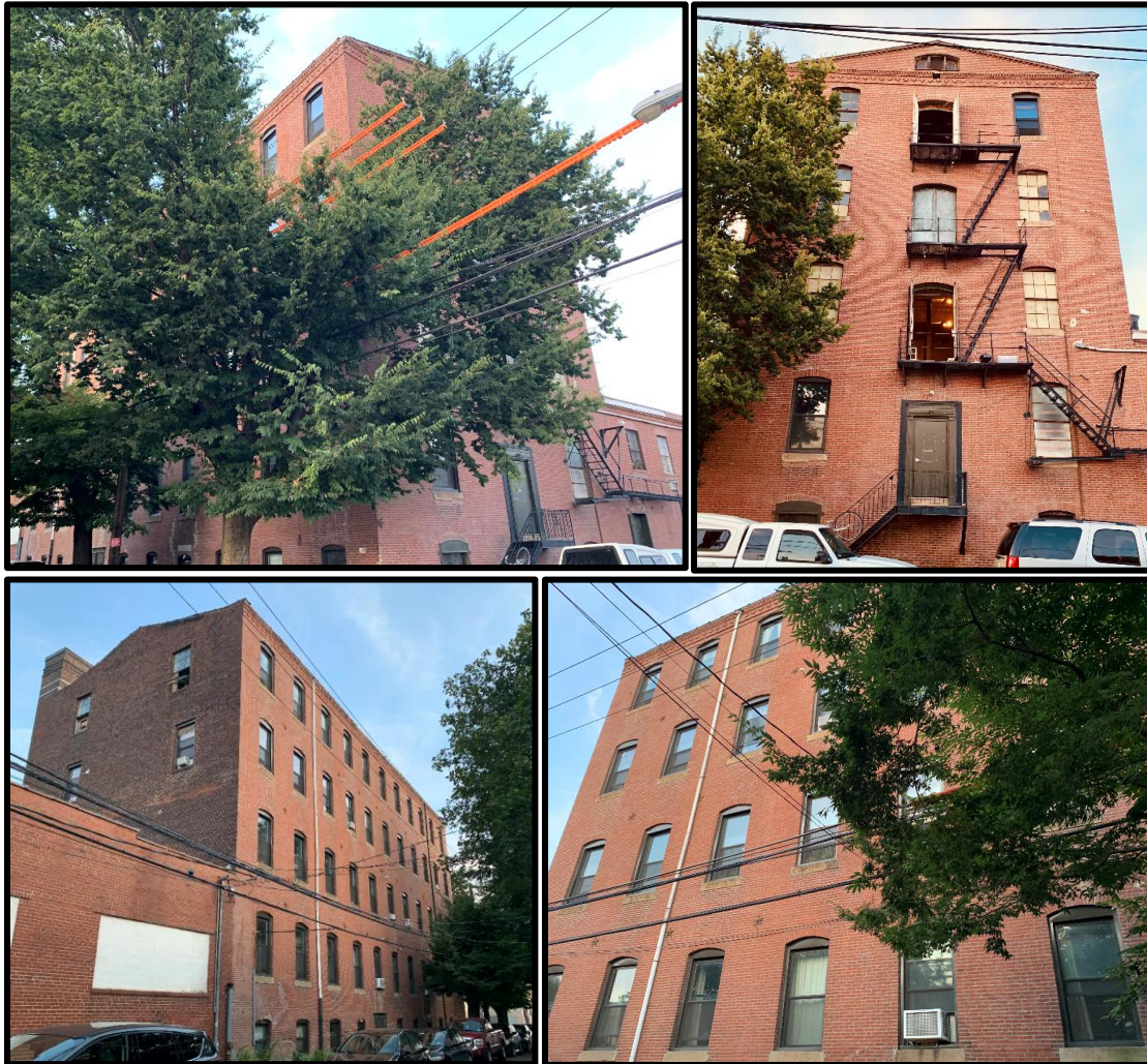
Figure 8. Top left: The southwest corner of Building 1. Figure 9. The south elevation of Building 1. Figure 10. Bottom left: The north and west elevations of Building 1. Figure 11. Bottom right: The west elevation of Building 1. Source: Oscar Beisert, 2019.
