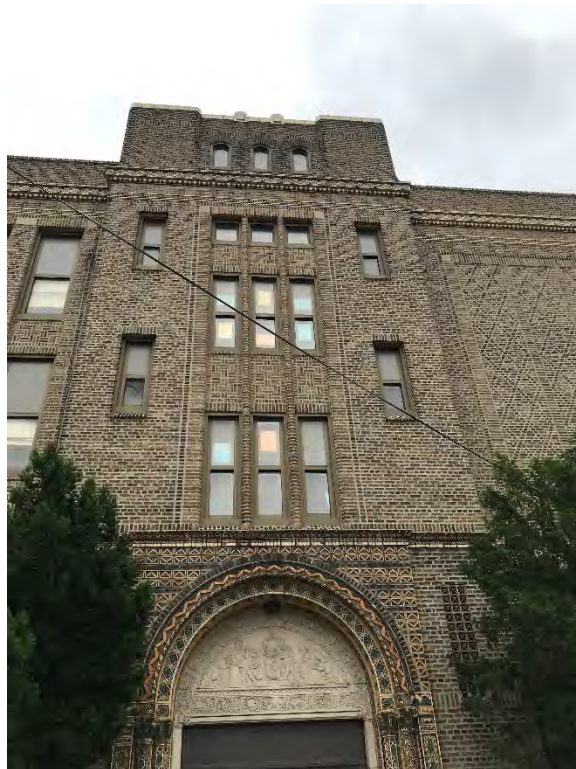
Photo 4 – North Elevation (right side) – 3/A-201
