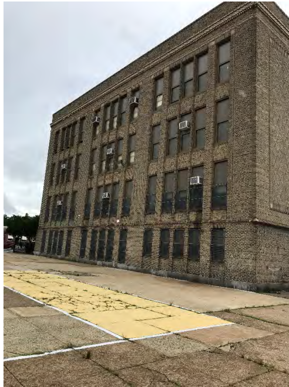
Photo 3 – West Elevation – 2/A-201
