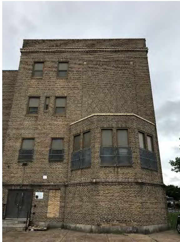
Photo 1 – South Elevation (right side) 3/A-202
