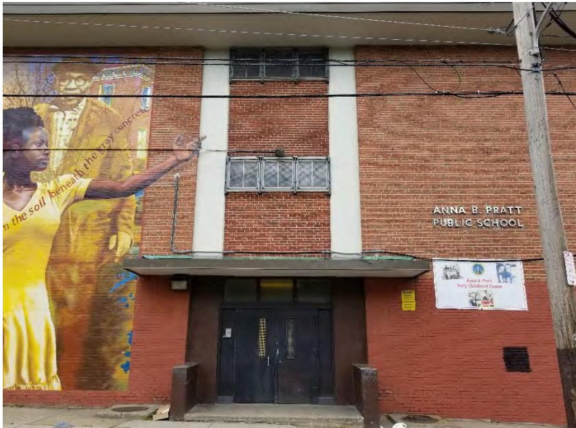
Detail of Existing Main Entry Doors and Frames
