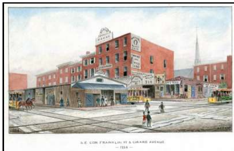
Figure 27. View of the market sheds in 700 block of Girard Avenue in 1884. Source: B.R. Evans, “S.E. Cor. Franklin St. & Girard Avenue, 1884,” Library Company of Philadelphia.
