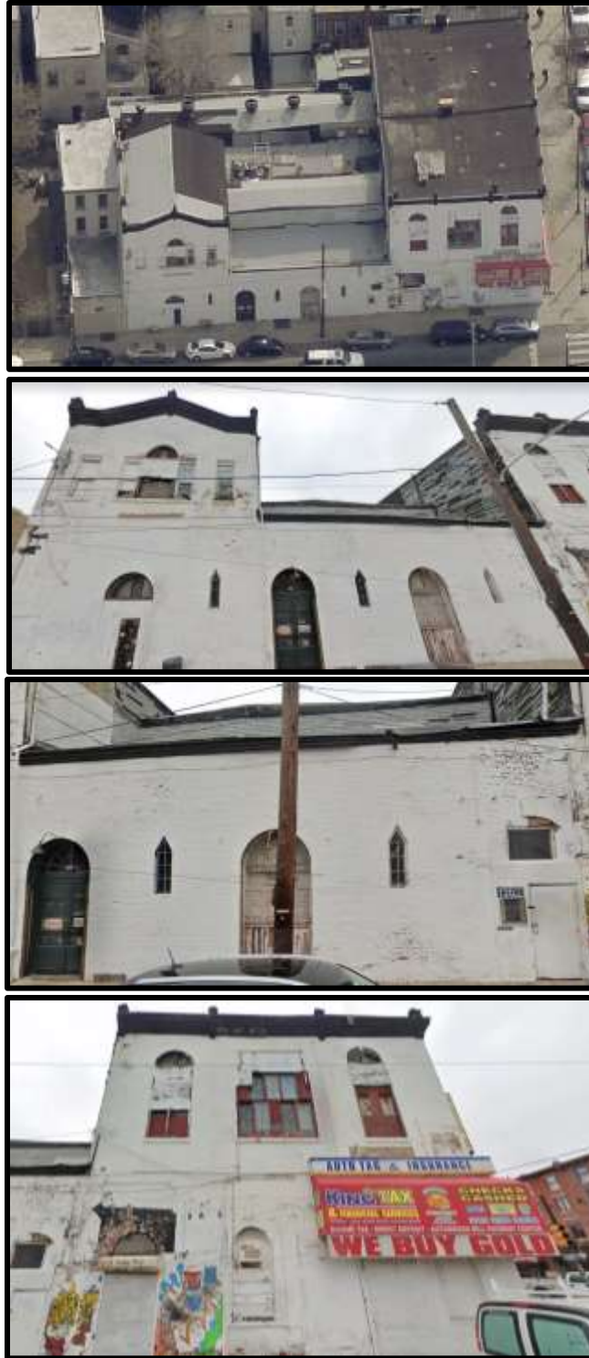
Figure 8. Top: Looking east at the side (west) elevation of the subject property. Source: Pictometry, Atlas, City of Philadelphia, 2019. Figure 9. Upper middle: The side (west) elevation of the Rear Hall. Figure 10. Lower middle: The side (west) elevation of the Market Shed. Figure 11. Bottom: The side (west) elevation of the Headhouse. Source: Google.
