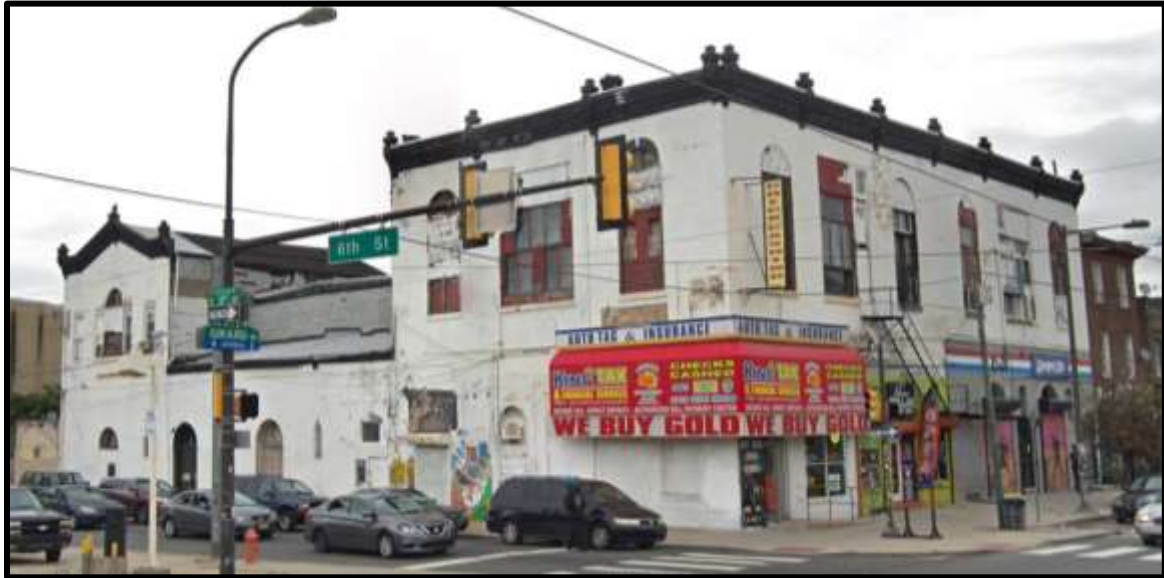
Figure 3. The side (west) and the primary (south) elevations. Source: Google.
