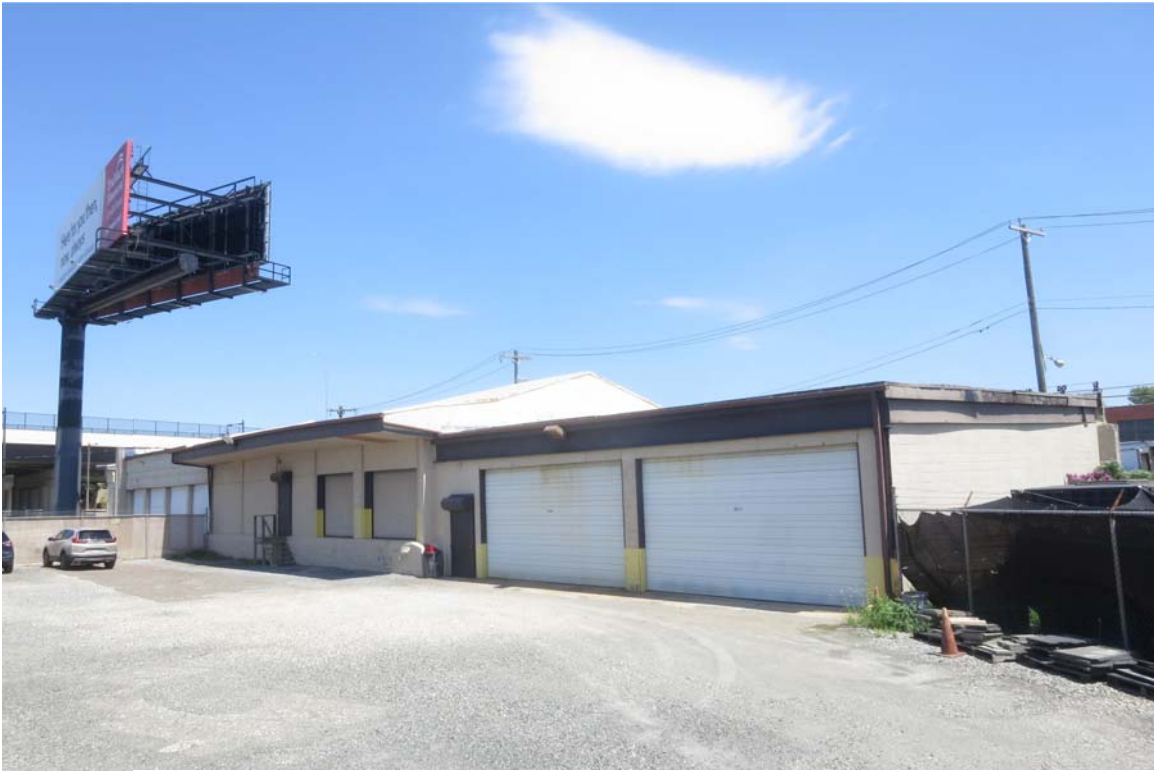
1615 N Delaware Ave Buildings looking form the rear of property
