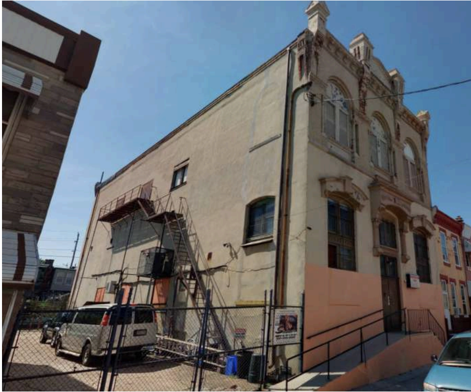
Figure 4: South (side) and west (front) elevations (Cyclomedia/Philadelphia Atlas)
