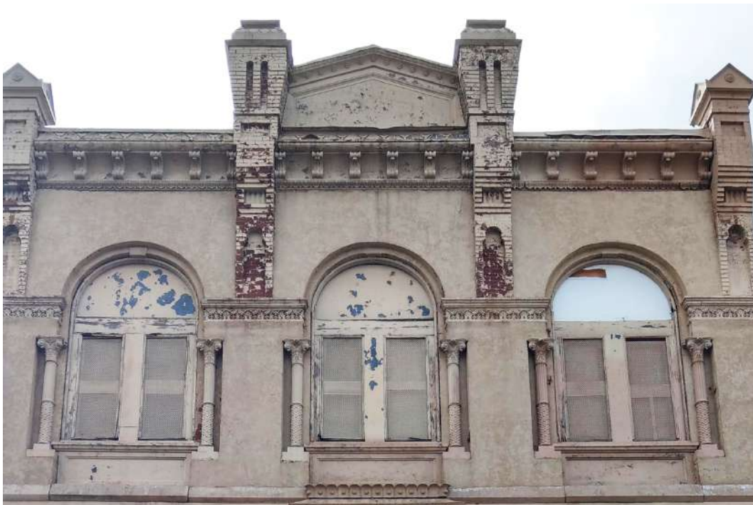
Figure 3: West elevation detail
