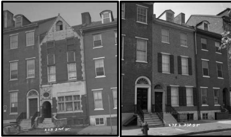
Figure 39. Left: The house at 238 S. 3 rd Street in 1961 with a once-fashionable revivalist façade, showing the use of a gable to disguise the earlier dwelling. Figure 40. Right: The same house at 238 S. 3 rd Street in 1964 after the revivalist façade was removed and the earlier appearance restored. Source: Philadelphia Historical Commission.
