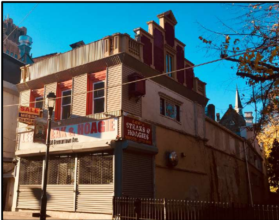
Figure 18. The primary (northeast) and northwest elevations of the Main Block, the 1857 Rear El, etc. Source: Oscar Beisert, 2019.
