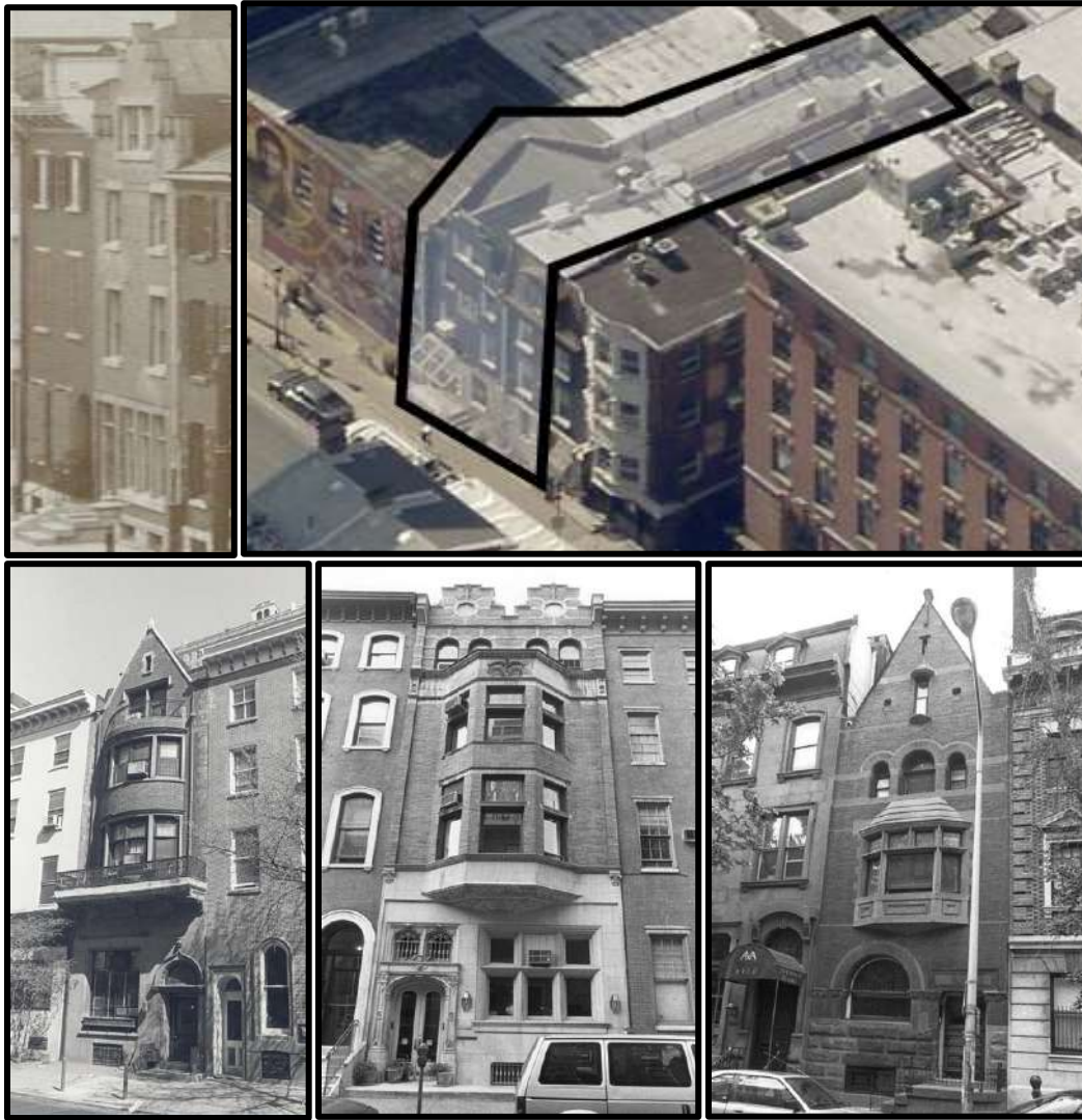
Figure 41. Top left: the Henry Minton House, S. 12 th Street, was refaced in the 1890s to conceal the earlier, outdated appearance of the building, employing a simple stepped gable to connect the old dormer opening and roofline to the new façade. Source: Free Library of Philadelphia. Figure 42. Top right: A profile view of the Henry Minton House, showing how the stepped gable was used to create a new façade, but also retain the entire structure of the earlier house. Source: Pictometry, Atlas, City of Philadelphia. Figure 43. Left: The design of 1721 Spruce Street employs a central gable to distinguish the building from its Italianate neighbors. Philadelphia Historical Commission, 1986. Bottom middle: The design of 1822 Spruce Street employs a stepped gable to distinguish the new façade or building from its earlier Italianate neighbors. Source: Philadelphia Historical Commission, 1995. Figure 44. Bottom right: The design of 1922 Spruce Street uses a gable or parapet to make the building stand out from the earlier Victorian houses in the 1900 block of Spruce Street.
