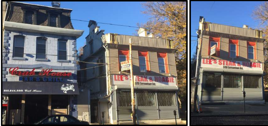
Figure 16. Left: The primary (northeast) and southeast elevations of the Main Block of the subject property. Figure 17. Right: The primary (northeast) elevation of the Main Block subject property. Source: Oscar Beisert, 2019.
