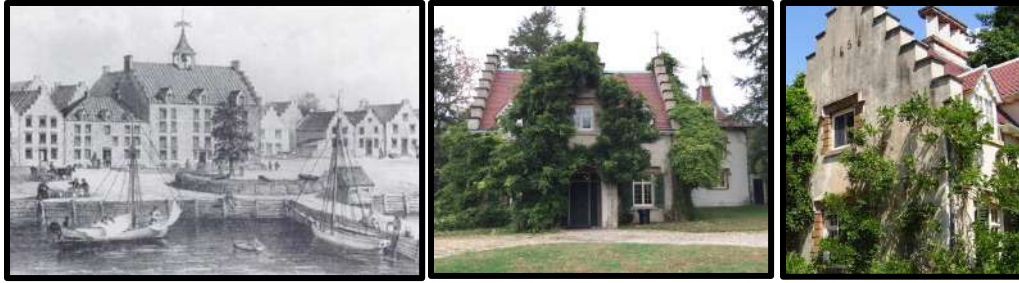
Figure 36. Left: Stadt Huys (City Hall) in 1641–42, New Amsterdam (New York City), New York. Source: Gelernter, Mark. A History of American Architecture: Buildings in Their Cultural and Technological Context . (UPNE, 2001), 50. Figure 37. Middle: Sunnyside, the home of Washington Irving in the Hudson Valley, New York. Like the subject property, Irving expanded upon an earlier house to create his Dutch or Flemish Revival style house. Source: Splorers Weekly. Figure 38. Right: A detail of a stepped gable end at Sunnyside. Source: Beyond My Ken (website).
