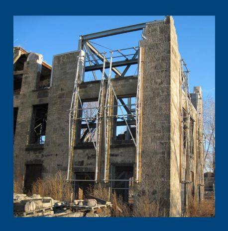
Stabilizing masonry after decades without a roof
