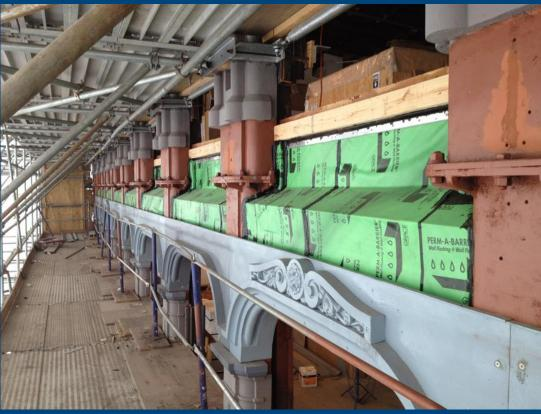
Scaffolding used to provide external lateral bracing
