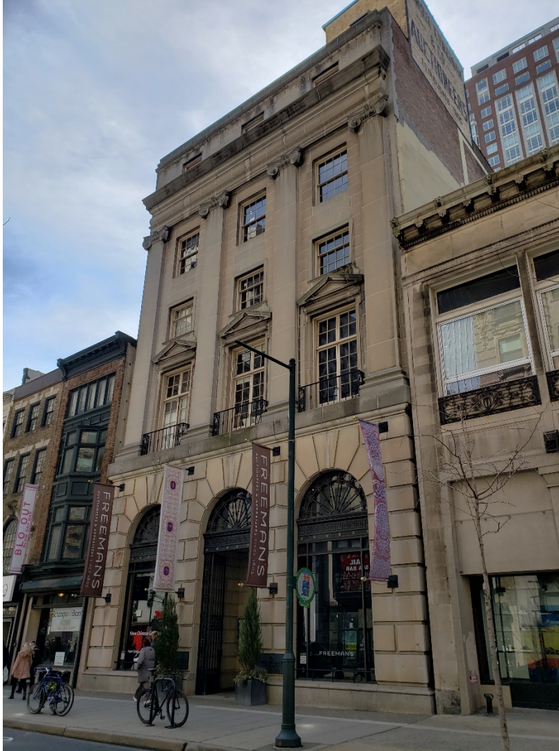
Figure 2. Chestnut Street façade, 2018. (Source: Philadelphia Historical Commission)
