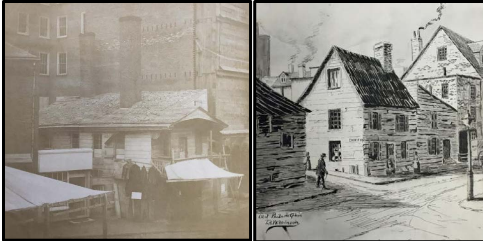
Figure 7. Left: The Loxley House, one of the most famous of the early wooden houses of Philadelphia. Notice that the house is essentially like a half house front gable disguised by a projecting gable-front porch roof. Figure 8. Right: Similar to the building type that is the subject of this nomination, the wooden house at the northeast corner of Cherry and Darien Streets in Center City. This drawing is by T.H. Wilkinson. Source: Castner Scrapbooks, Free Library of Philadelphia.
