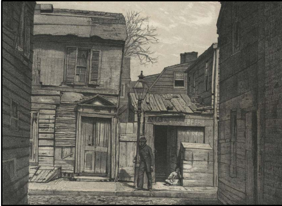
Figure 25. Seen between a variety of wooden houses, the Georgian doorway (on left) in the lithograph is a representative of the Georgian vernacular that pervaded the architectural landscape of Philadelphia, even in the largely unknown context of frame buildings in what reads as the Quaker City. Adjacent, in the foreground, as well as the background, and on right are all manner of timber frame houses—one even prominently displays the lines of a Gambrel roof. This scene is, on a whole, a court of frame dwellings, depicted in The little homeless one or "no one to kiss me good night," a lithograph by P.S. Duval, Philadelphia, dated 1867. Source: Library Company of Philadelphia.
