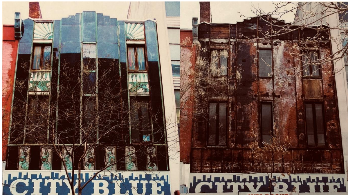
Figure 2: Comparison of the 1106 Chestnut Street façade just before and immediately following the removal of the glass and metal panels. Source: Philadelphia Historical Commission.
