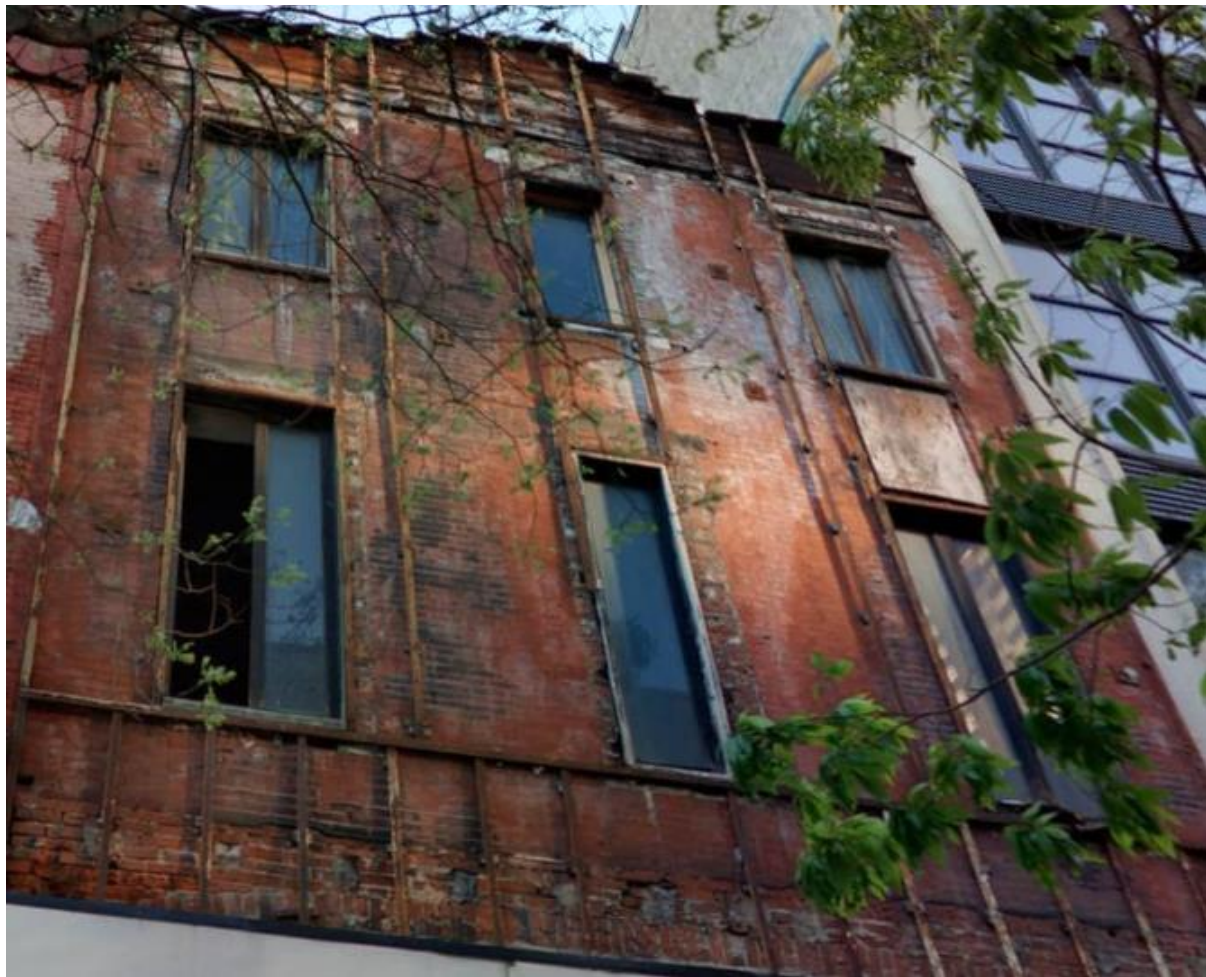
Figure 4: Portion of the 1106 Chestnut Street façade where the glass and metal panels were removed, May 2020. Source: Cyclomedia.
