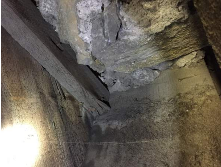
Corner masonry infills supported by timbers at the Lower Bell level
