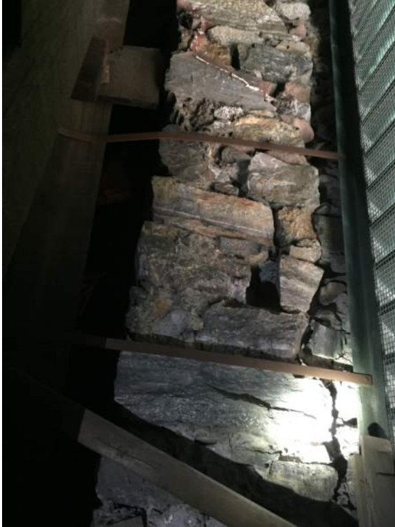
Note smaller stones, lack of mortar
