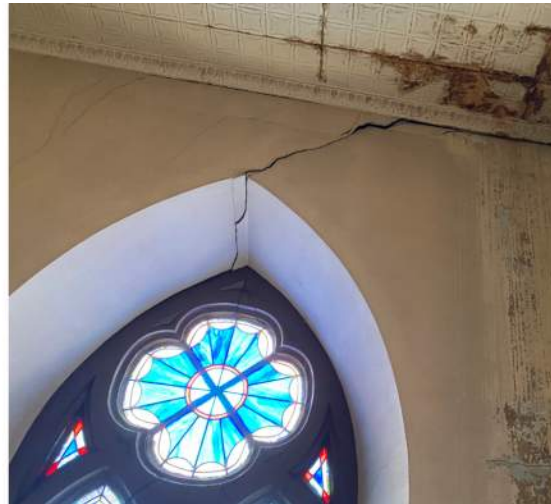
Northern wall eastern tower below mid-level (wood window frame cracked)
