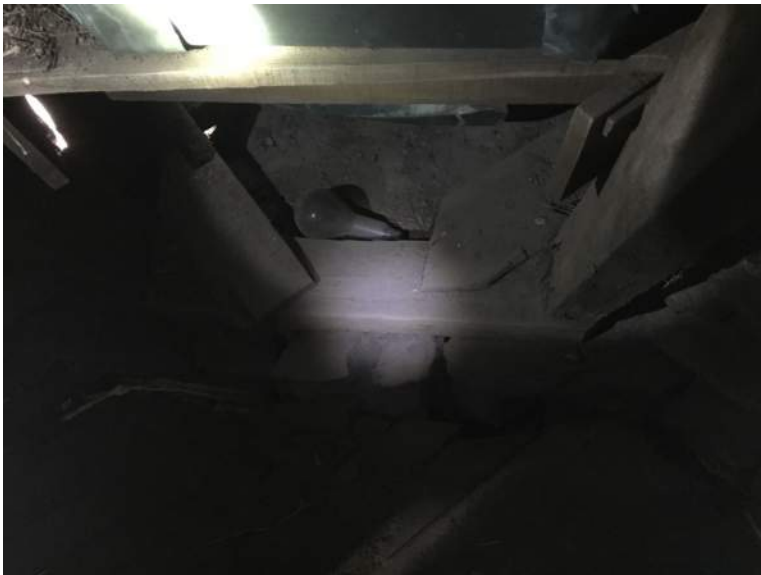
Corner steeple support supported on corner masonry infills
