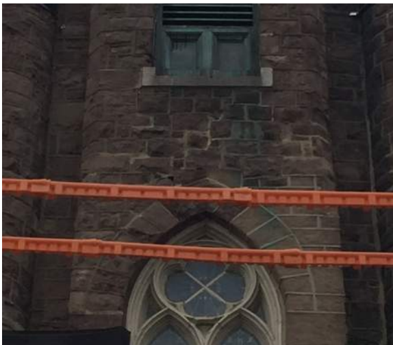
Eastern wall eastern tower below mid-level (wood window frame cracked)
