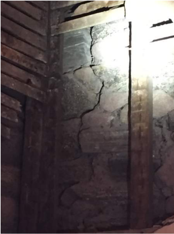
INTERIOR THROUGH CRACK – CHOIR TO MID-LEVEL NE TOWER
