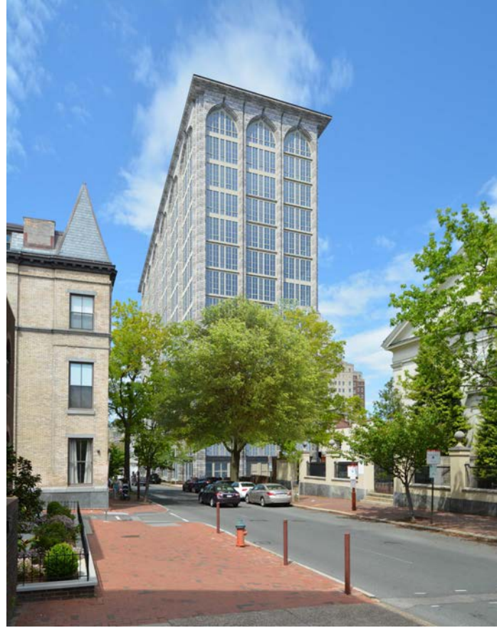
View From 3rd Street Looking North
