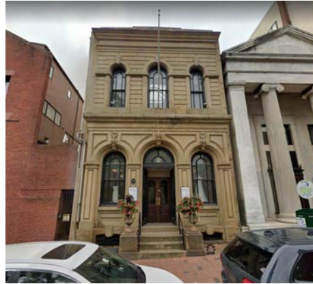
Context - 3 Window Bays at 304 Walnut Street
