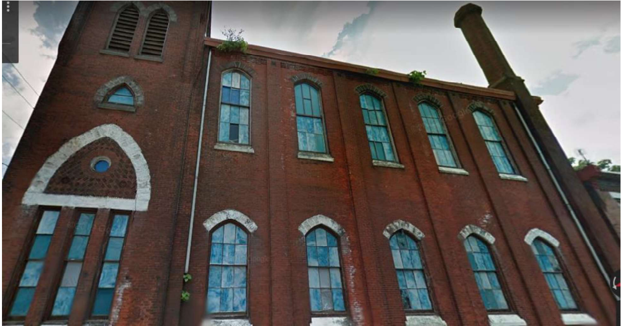
Figure 2: The west side (S 18th St) elevation of 1730 Wharton in 2011, showing the historic marbled blue glass windows in their original configuration.
