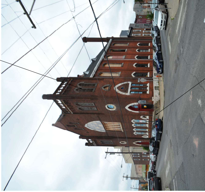
Proposed: Removal of Fake Vents -Replace with New Windows
