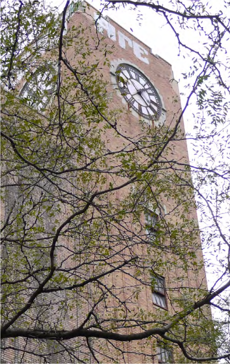
Figure 10. Detail view of clock tower from the southeast.
