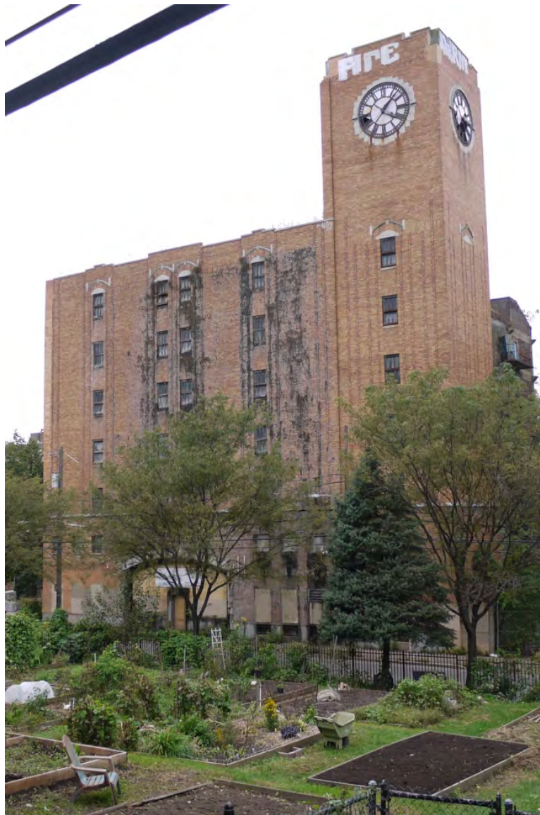
Figure 2. Southeast façade of 237 - 253 East Church Lane.
