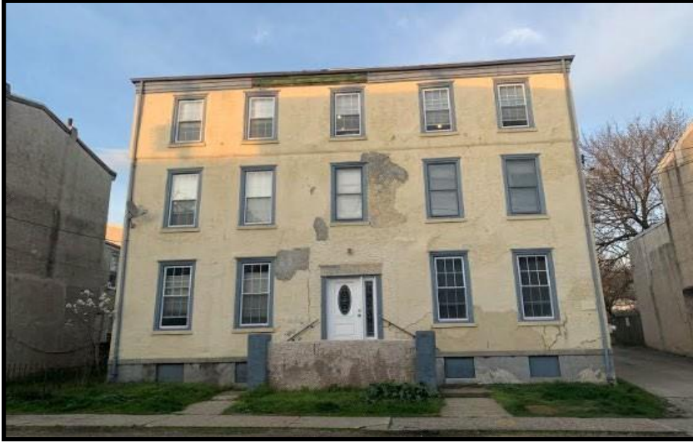
Figure 7. The primary (southwest) elevation of the Levering-Smick-Arbuckle House. Source: Oscar Beisert, 2020.
