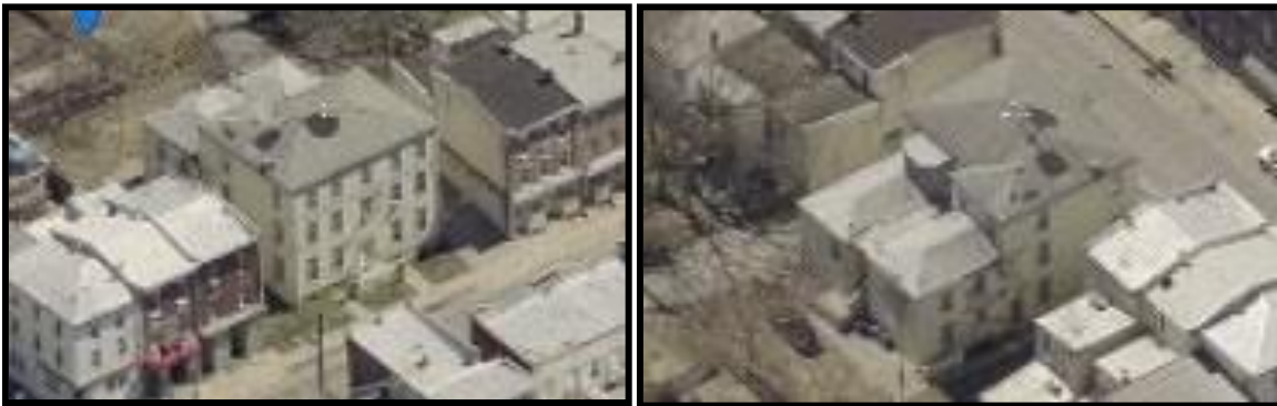
Figure 5. Left: Looking south at the primary (north) elevation of the subject property. Figure 6. Right: Looking north at the rear (south) elevation of the subject property. Source: Pictometry, Atlas, City of Philadelphia, 2019.
