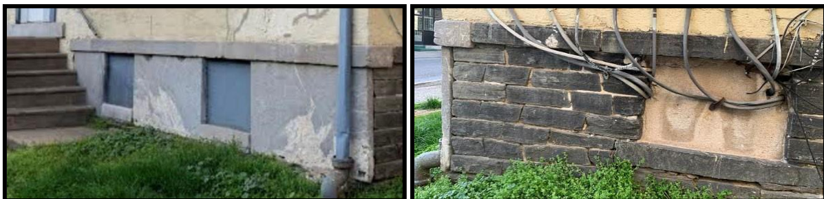
Figure 8. Left: The marble basecourse and facing at the basement level, as well as the infilled windows therein. This view also shows the marble threshold on left at the base of the primary entrance. Figure 9. Right: The stone foundation at the side (southeast) elevation, also showing an infilled basement window. Source: Oscar Beisert, 2020.
