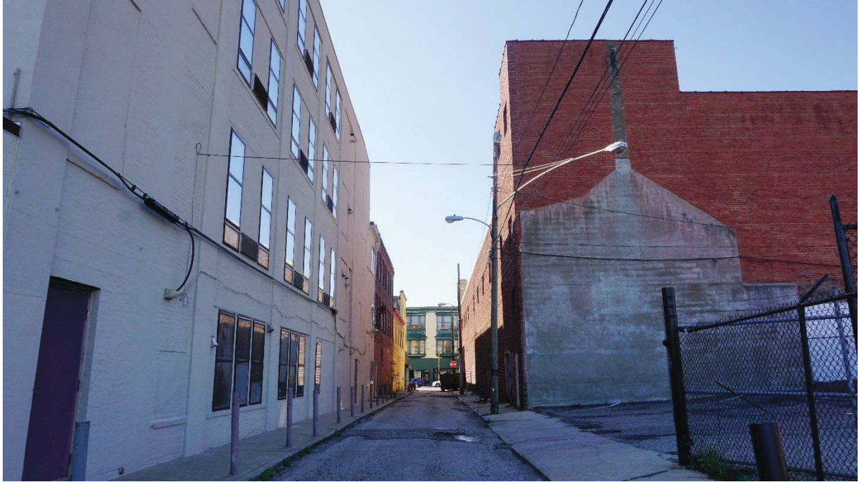
Figure 8 View of the rear façade of the building and out to Germantown Avenue from E. Woodlawn Street November 2019. Photo by Author.
