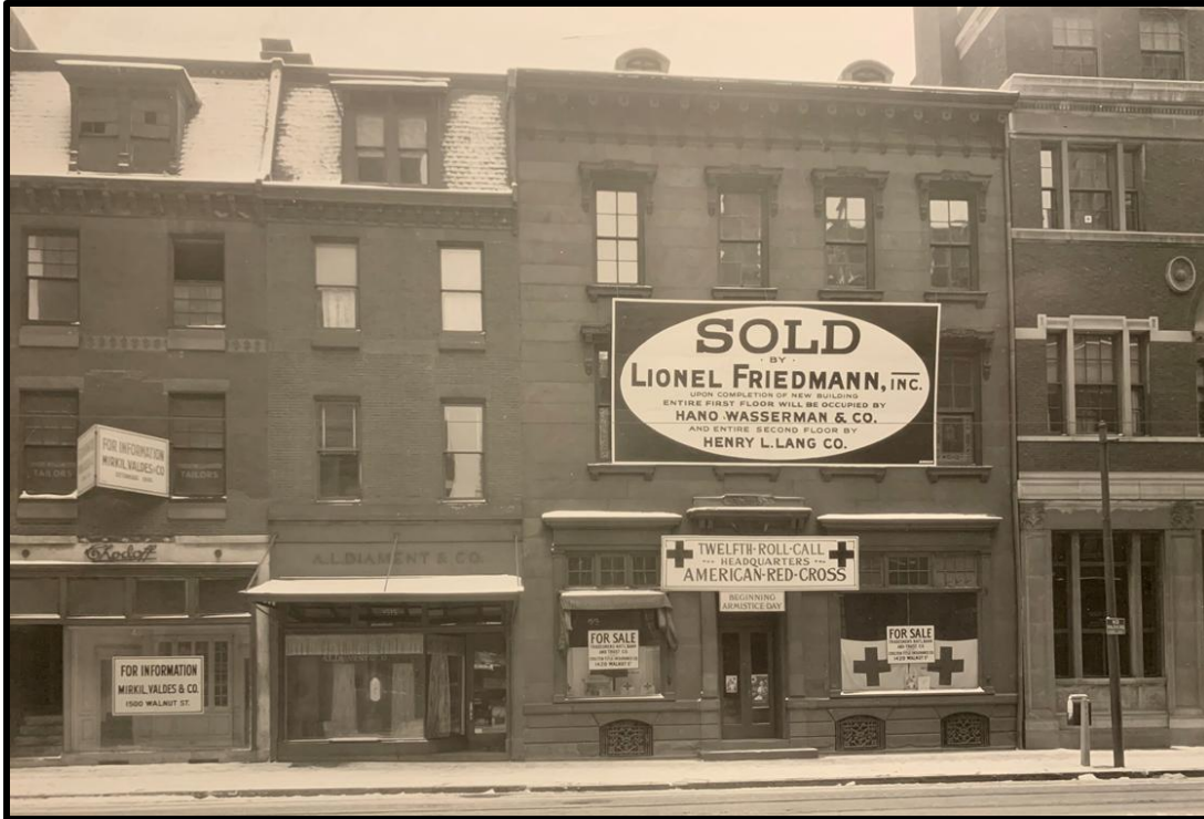
Figure 16. This photograph of the subject property in 1928 shows the original building prior to its demolition with a sign announcing that Hano, Wasserman & Co. would soon occupy the site. Source: Walnut Street Files of the Penrose Collection – Photographs, The Historical Society of Pennsylvania (HSP).
