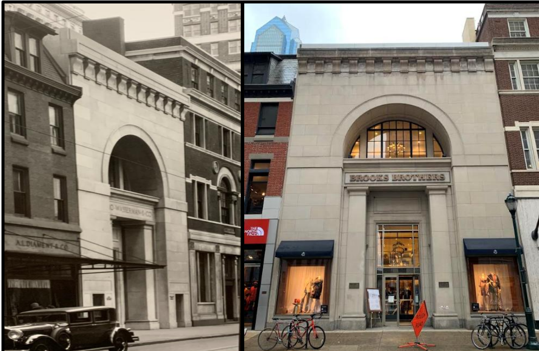
Left: Figure 1a. A view of the subject property just after it was built in October 1930. Source: Walnut Street Files, Penrose Collection – Photographs, the Historical Society of Pennsylvania; and Right: Figure 1b. The south elevation of the subject property. Source: Oscar Beisert, 2019.
