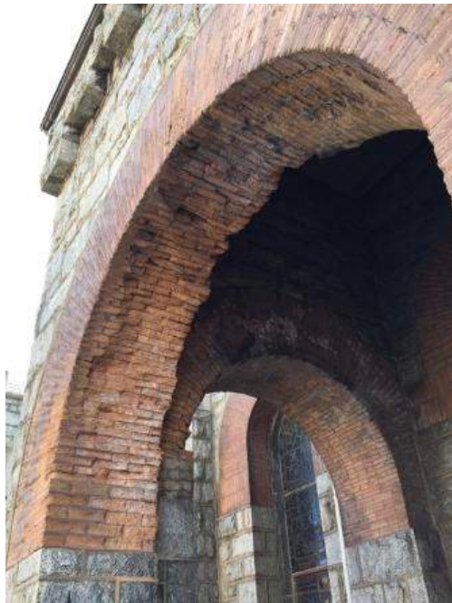
Figure 11. Visible deterioration of the brick arch on the underside of the northern façade's loggia [Kevin Block, November 2019].
