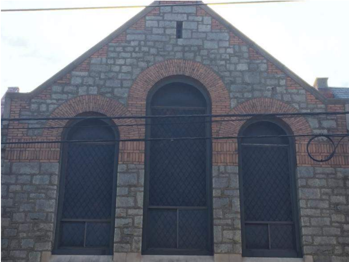
Figure 4. The Roman brick arches and banding on the western (principal) façade, as well as the stepped gable ornamental brickwork [Kevin Block, November 2019].
