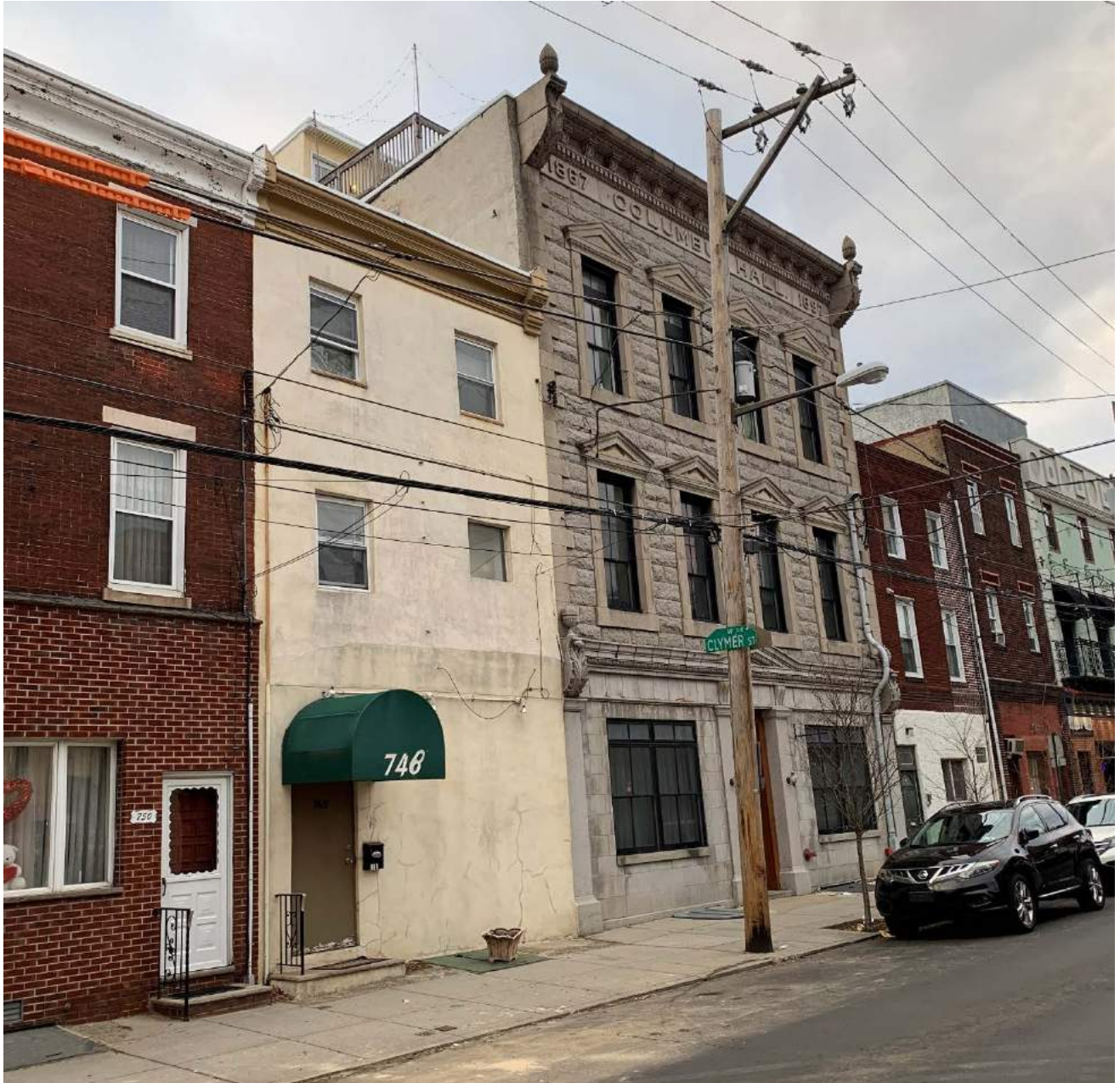
View showing rooftop addition and deck, January 2020.
