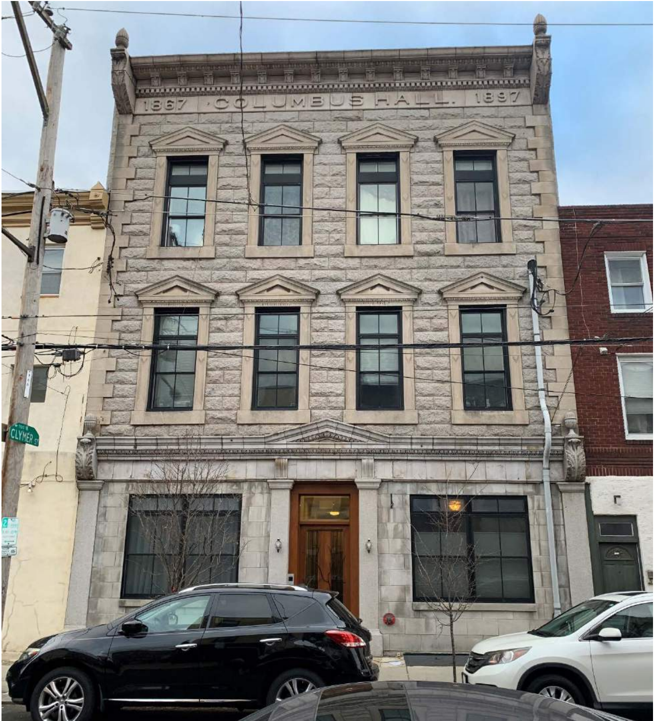
Primary (east) façade, January 2020.
