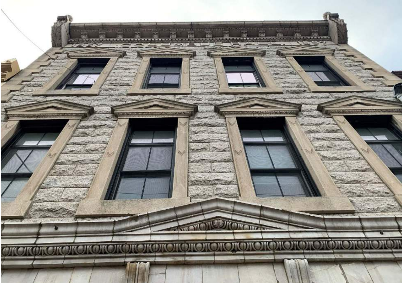
View looking up from entrance to cornice, January 2020.
