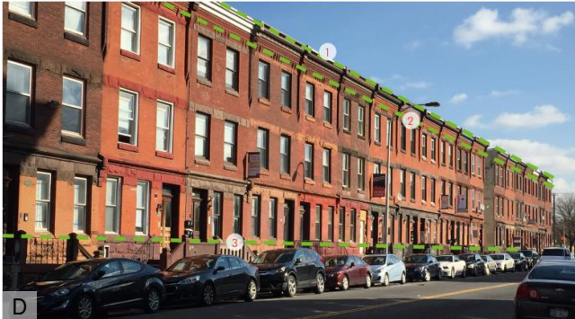
D 1600 Block of Diamond Street, North Side 1. Urban fabric establishes a horizontal datum. 2. Cornice datum. 3. Base datum typically including a stoop at each dwelling.
