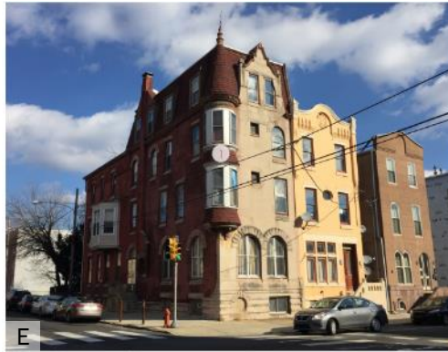
E 1831-1835 Diamond Street 1. Articulated corner.
