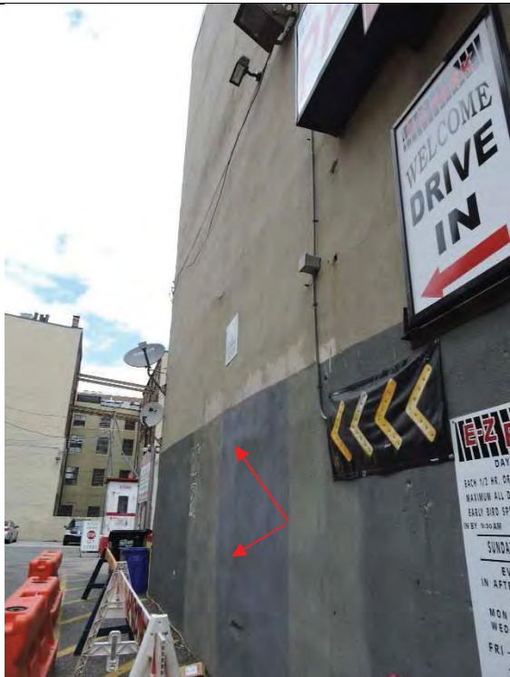
Stucco and wall are buckling.
