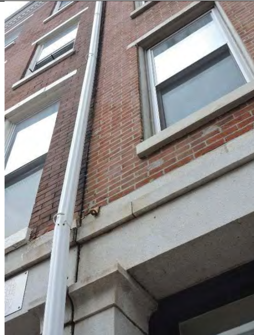
Full height joint between the facades.
