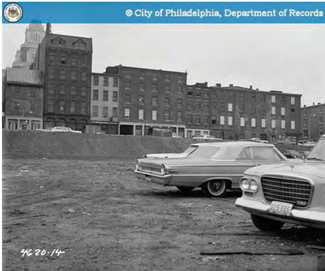
Demolition of Delaware Avenue and Water Street buildings providing view of Front Street, looking west in trench for I-95: Photograph: Department of Records, Larry Williams, 1966. Note no retaining walls and simple grading between Front Street and the future site of the expressway.
