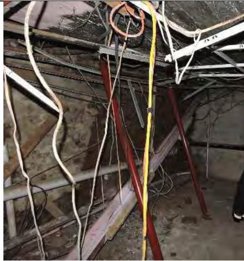
Screw jacks under the unsupported joists fell over recently.
