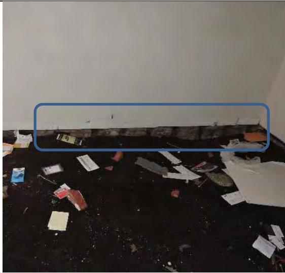
First floor joists have fallen out of the bearing pockets.
