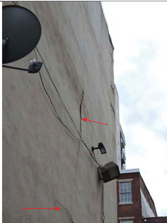
Stucco is delaminating.
