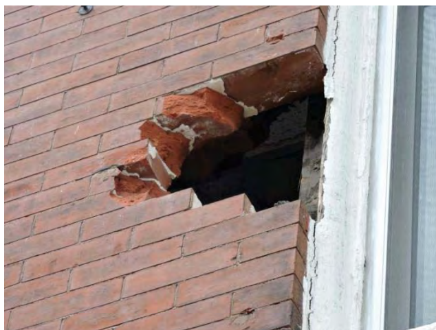
Left: Detail of south façade 107 Chestnut Street, showing failure of middle left pier of the front wall adjacent to second floor window, photograph, Fred Baumert, Keast & Hood, May 11, 2020.; Right three wythes of brick, two inner layers of salmon brick filling out wall to depth of window frame with outer pressed brick facing Chestnut Street. The collapse suggests failure of a bond course in the salmon brick between the layers (or this may have been where the mason laid cut brick ends); photograph, Fred Baumert, Keast & Hood, May 11, 2020.
