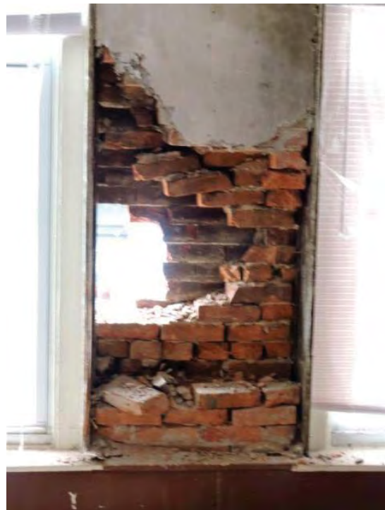
Left: Detail of south façade 107 Chestnut Street, showing failure of middle left pier of the front wall adjacent to second floor window, photograph, Fred Baumert, Keast & Hood, May 11, 2020.; Right three wythes of brick, two inner layers of salmon brick filling out wall to depth of window frame with outer pressed brick facing Chestnut Street. The collapse suggests failure of a bond course in the salmon brick between the layers (or this may have been where the mason laid cut brick ends); photograph, Fred Baumert, Keast & Hood, May 11, 2020.
