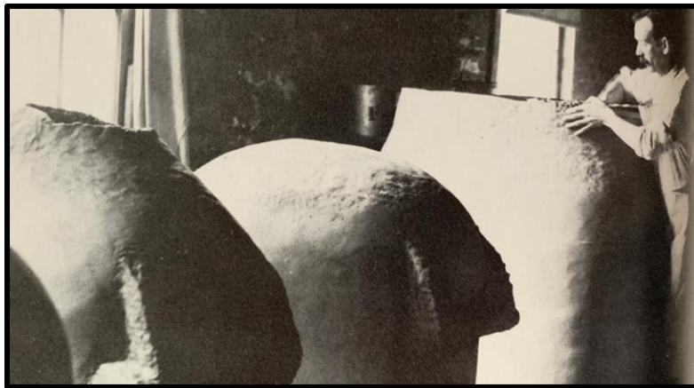
Figure 42. An employee of Gillinder & Sons engages in the potmaking step of the manufacturing process. Source: Scranton, Philip, and Walter Licht, Work Sights, Industrial Philadelphia, 1890–1950 , (Philadelphia: Temple University Press, 1986), 75–77.
