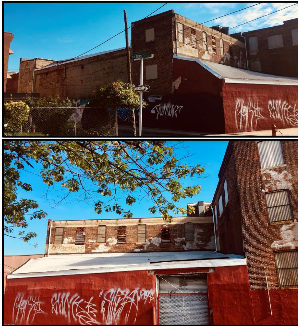
Figure 8. Top: The west elevation of the Buildings 2: Stable and 3: Shed Addition. Figure 9. Bottom: The south elevation of the Buildings 2: Stable and 3: Shed Addition. Source: Oscar Beisert, 2019.
