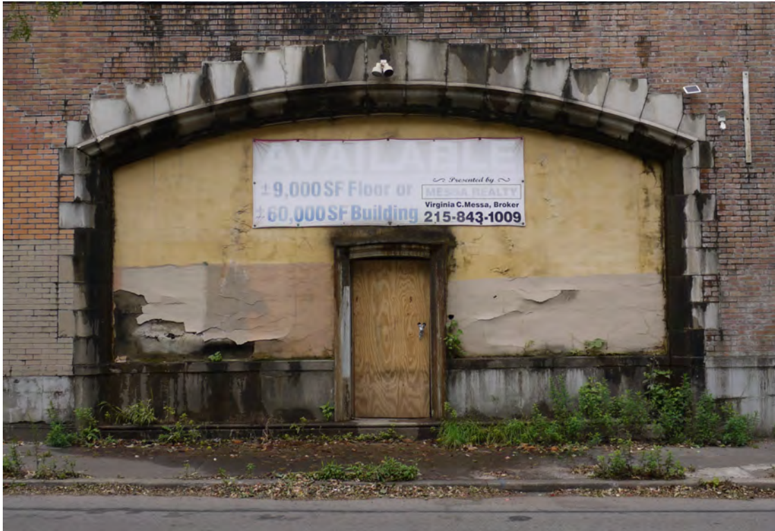
Figure 9. Detail view of the entrance on the southeast façade of the Germantown Fireproof Storage Company building.
