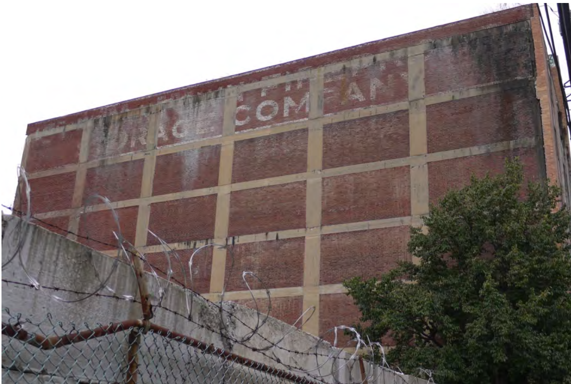
Figure 3. Detail view of southwest elevation.
