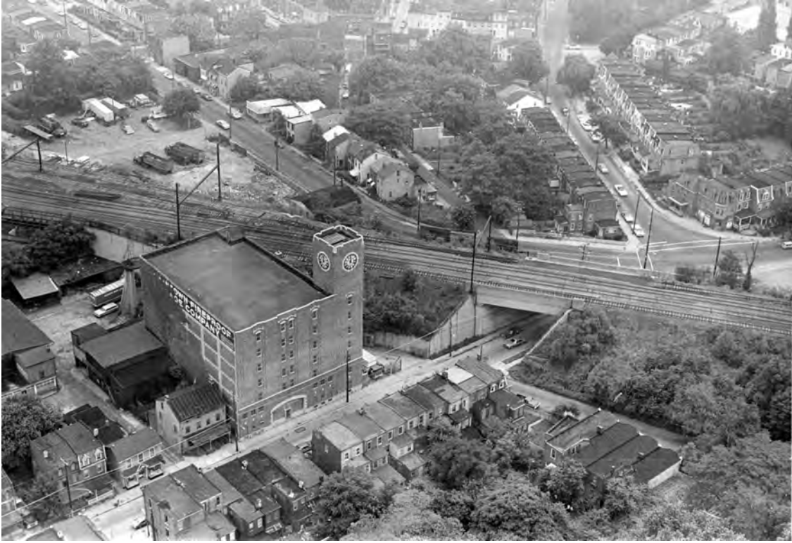
Figure 11. Aerial view of Germantown Fireproof Storage Company, 1931. Germantown Historical Society.
