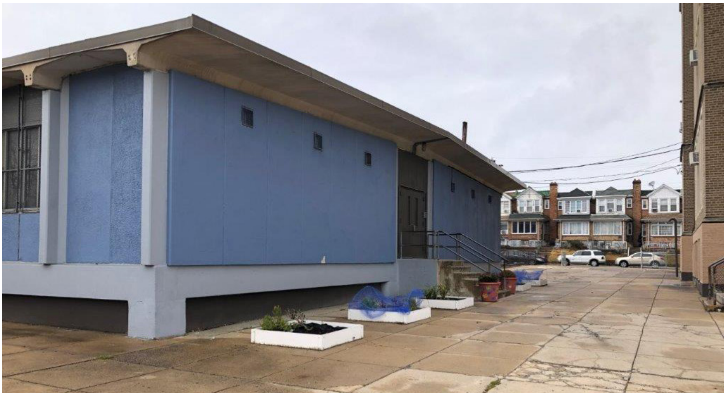
PHOTO 1: Existing Planters at Pre-K Building; Location of 'Early Action' Project by Mural Arts & Community Members
