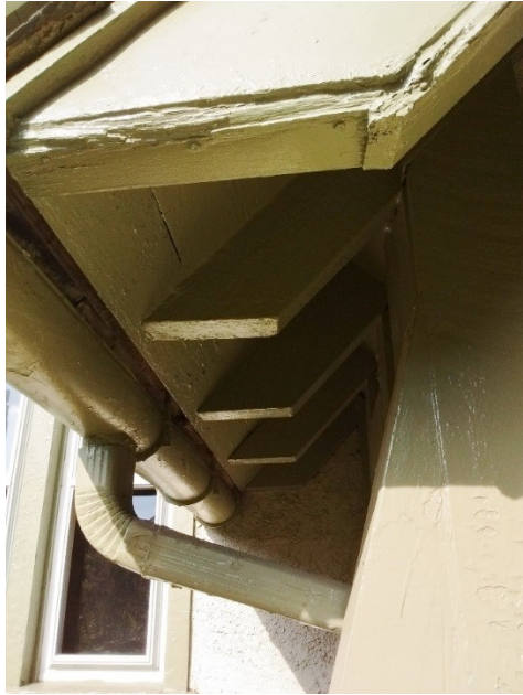
Figure 7: Exposed rafters in unenclosed eave. Steven Peitzman, August 2019.
