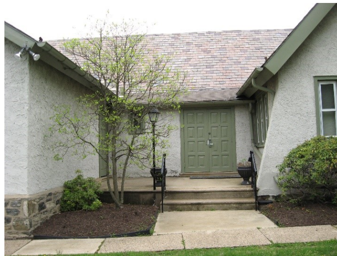
Figure 13: West view of 1938 addition. Steven Peitzman, June 2019.
