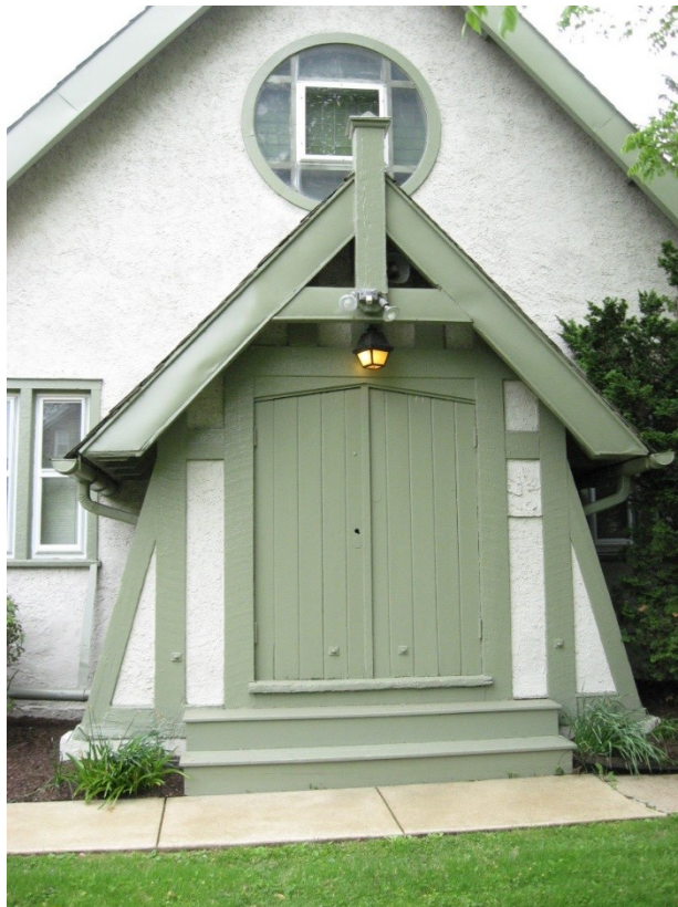
Figure 6: West-facing porch. Steven Peitzman June 2019.
