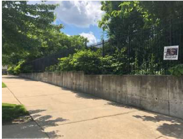
Lot B Retaining Wall
