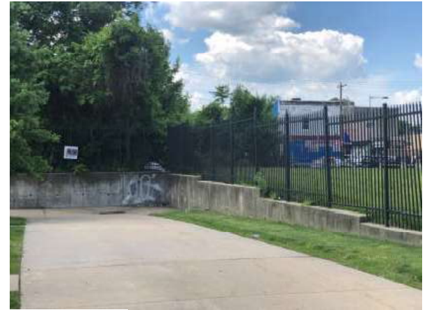
Lot B Retaining Wall
