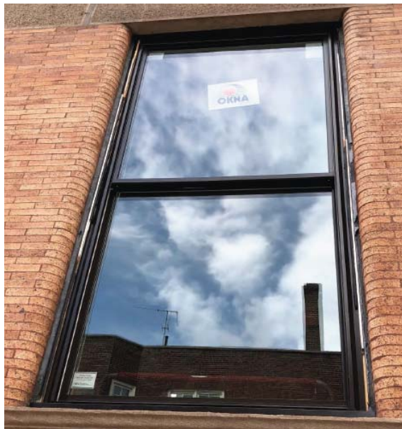
Figure 3: Left, a replacement basement window, with non-historic infill at the top. Right, a typical upper-floor window pre-frame panning.
