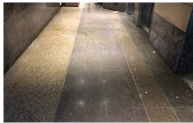
5. TERRAZZO FLOOR PATTERN WITH BRASS TRANSITION STRIPS
