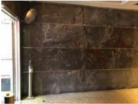
2. ORIGINAL MARBLE CLADDING WITH METAL STRIPS
