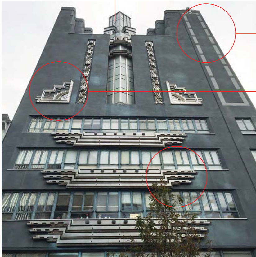
LEFT: STEEL AND BRONZE SPANDREL PANELS INSTALLED IN THE EARLY-MID 80S TO REPLICATE ORIGINAL DESIGN
