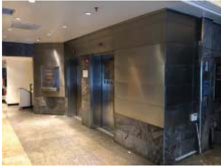
3. METAL PANEL WALL CLADDING FLUSH WITH ADJACENT ORIGINAL MARBLE PANELS BELOW
