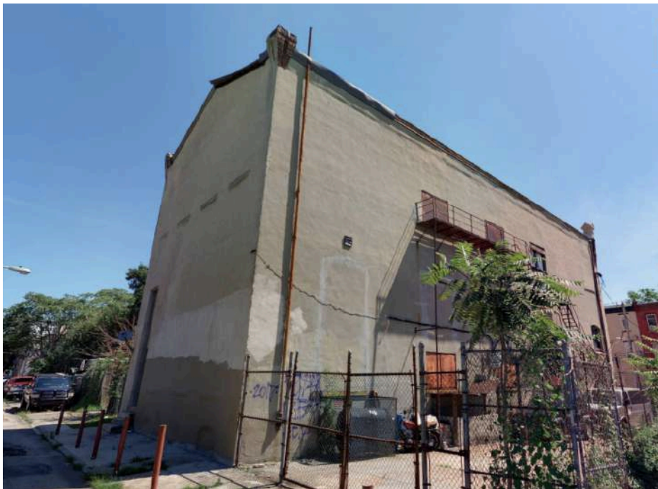
Figure 5: East (Leithgow Street) and south (side) elevations (Cyclomedia/Philadelphia Atlas)
