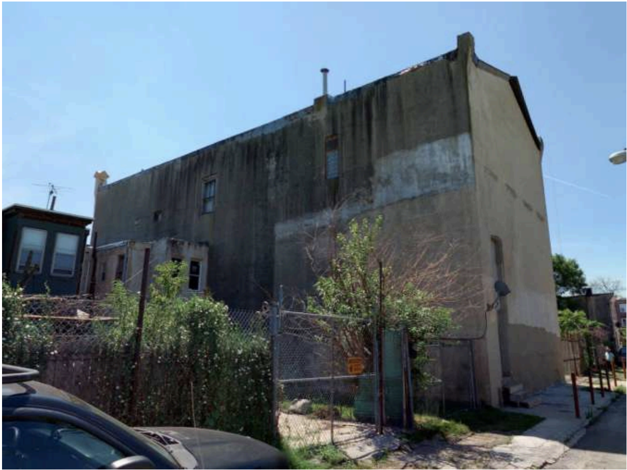
Figure 6: East (Leithgow Street) and north (side) elevations (Cyclomedia/Philadelphia Atlas)
