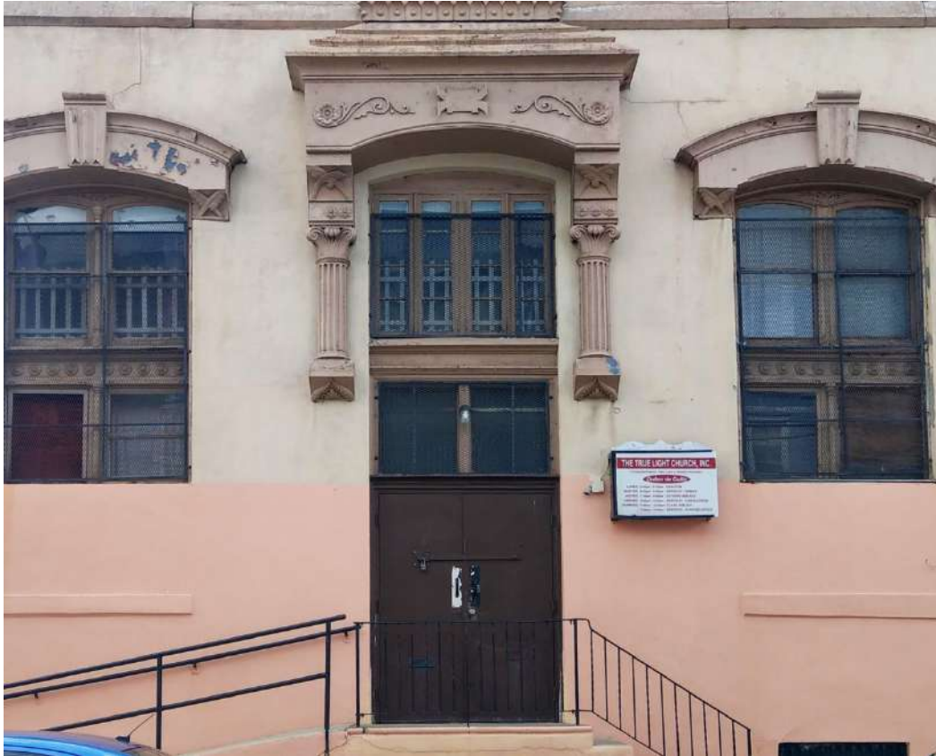
Figure 2: West elevation entrance detail
