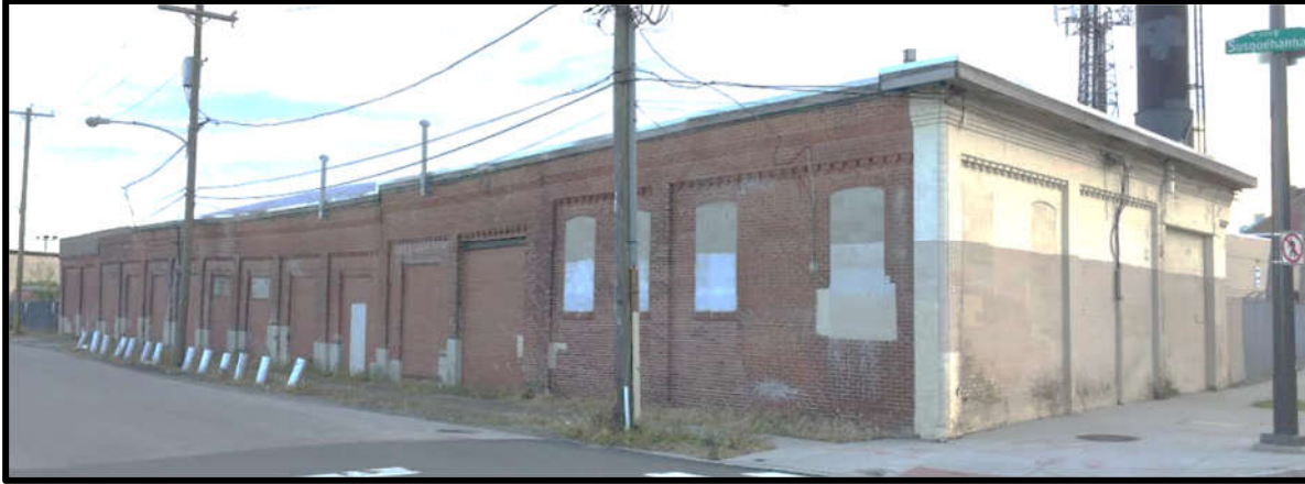
Figure 3. View from North Delaware Avenue at Susquehanna Avenue of the Empire Chain Works. Source: Oscar Beisert, 2019.
