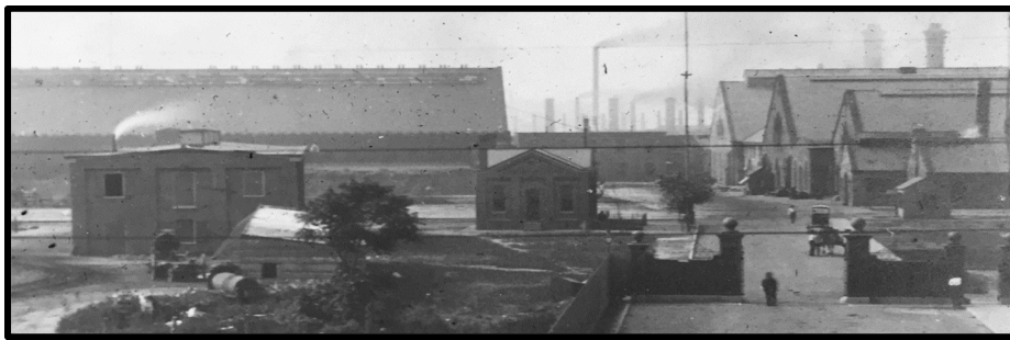
Figure 86. Looking north towards the Point Breeze Gas Works in c1899 with the original “Church Row” complex of sheds on right. Source: The PGW Photograph Collection, CAP.
