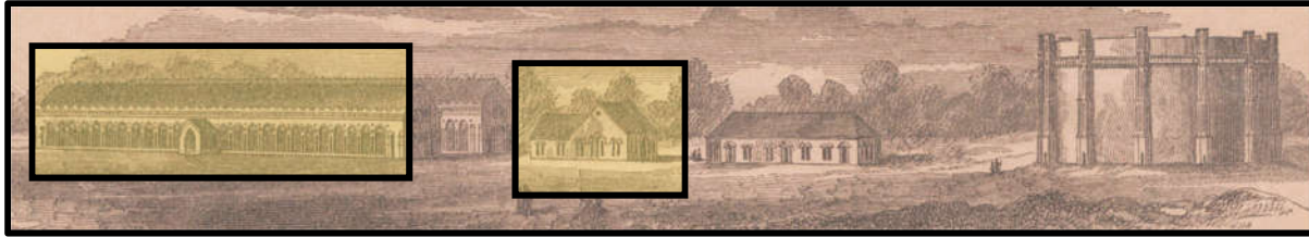
Figure 95. This early illustration shows the early buildings of the Point Breeze Gas Works, including Resource No. 1 (Figure 83): Purifying House (1853–54), highlighted in yellow at center. Also highlighted and outlined is a Retort House that features a façade defined by buttresses like Resource No. 3 (Figures 44 & 45): North Wall Ruins of Coal House (1855). Source: Twenty-Second Annual Report of the Trustees of the Philadelphia Gas Works to the Select and Common Councils of the City of Philadelphia, (January 1857), frontispiece. Source: The Library Company of Philadelphia.
