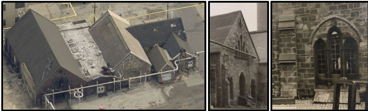
Figure 96. Left: looking southeast at Resource Nos. 1, 2, & 5. Source: Atlas, City of Philadelphia, 2018. Figure 97. Middle: The northeast elevation of Resource No. 2: Purifying House (1855), showing the Gothic Revival features shown below. Figure 98. Bottom right: A three-part lancet arch mullion window with colonettes exists within the confines of a projecting hoodmold or dripstone arch and a buttress with two tiers of stone coping. Source: The PGW Photograph Collection, CAP.
