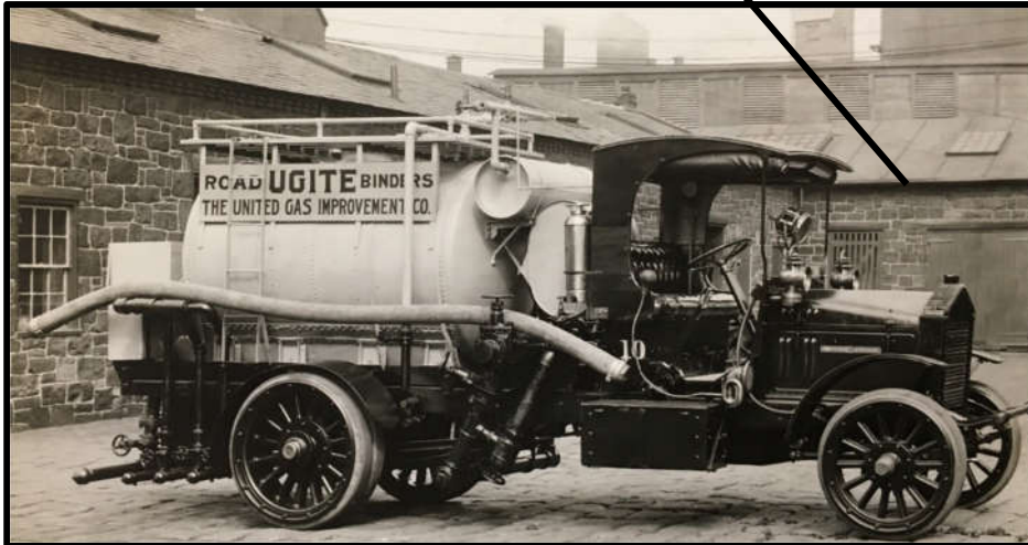
Figure 59. Top: Looking southwest at the side elevation of Resource No. 6: Shop (1859). Source: The PGW Photograph Collection, CAP. Figure 60. Center: Looking north at Resource Nos. 6, and 7, the primary elevations of which are circled in black and correspond with the image shown above. Source: Atlas, City of Philadelphia, 2018. Figure 61. Bottom: Looking northwest at the side elevation Resource No. 6: Shop (1859) as it connects to the back wing. Source: The PGW Photograph Collection, CAP.
