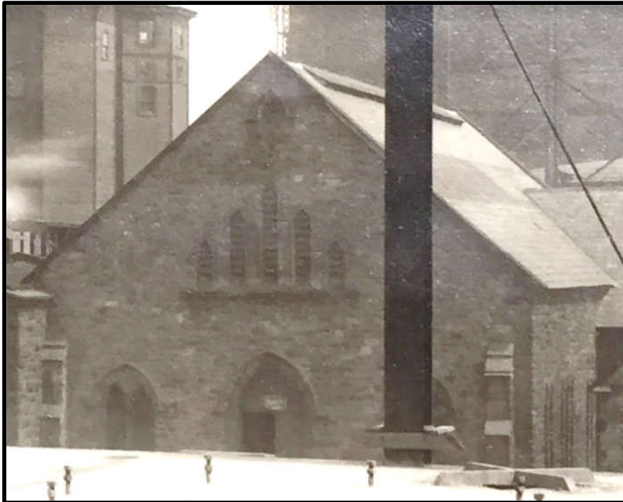
Figure 26. Top: The southwest elevation of Resource No. 2: Purifying House (1855). Source: Pictometry, 2019. Figure 27. Bottom: The northwest elevation of Resource No. 2: Purifying House (1855), dated 1910s. Source: The PGW Photograph Collection, CAP.
