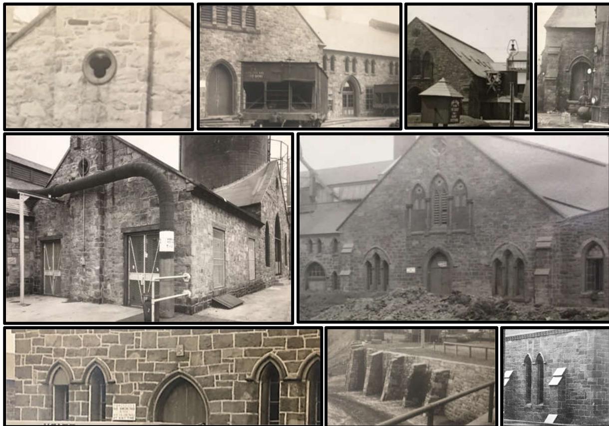
Figure 99. Top left: A trefoil opening in the primary (northeast) elevation of Resource No. 1a: Purifying House, Engine & Exhaust House (1853–54). Figure 100. Top middle left: Various apertures of Resource No. 5a: Purifying House (1859), showing various Gothic and lancet arch openings. Top middle right: Resource No. 5a: Purifying House (1859), showing the mullion window with colonettes. Figure 101. Top right: various openings in the Gothic Revival style. Figure 102. Middle left: Resource Nos. 1a and 1b, showing the various features of the Gothic Revival. Figure 103. Middle right: the northeast elevation of Resource No. 5a: Purifying House (1859) showing six lancet arch openings, a pointed Gothic doorway and a three-part mullion window defined by pointed arched openings, and a quatrefoil opening. Figure 104. Bottom left: The projecting hoodmolds and architraves of Resource No. 7: Shops (1859) set within the random ashlar façade. Figure 105. Bottom middle: The retaining wall at Resource 9: The Wharf (1859–99) with its stone buttresses. Figure 106. Bottom right: The image shows the two-tier buttresses with stone
