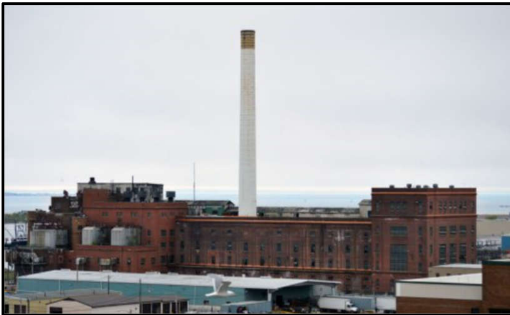
Bottom: New Bedford Gas and Light Company, 2015, which is pending reuse as part of a new aquarium. Source: Wikipedia.
