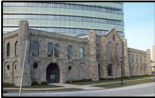
Buffalo Gas Light Company Works, built 1859, is preserved in Buffalo, New York as part of a corporate headquarters. Source: Wikipedia.
