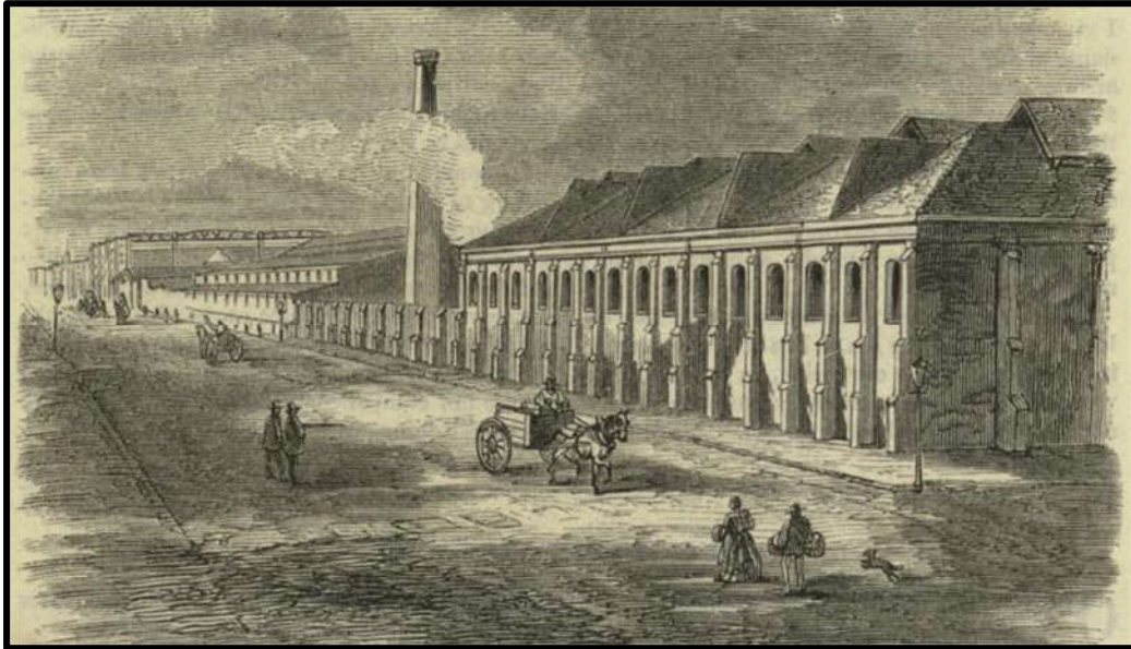
The Manhattan Gas-Works (Demolished), c. 1862. The company occupied the entire block between E. 15 and 16 Streets, Avenue C, and the East River. Source: NYPL Digital Collections.
