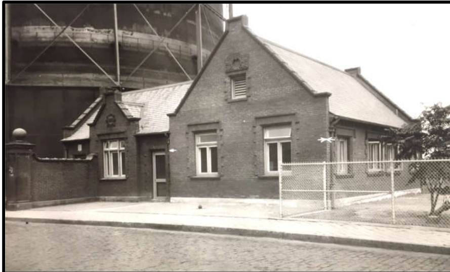
Figure 67. Top: Looking east at the primary (west) elevation of Resource No. 9a: U.G.I. Office & Dispensary (1899–1929). Source: Atlas, City of Philadelphia, 2018. Figure 68. Bottom: The southwest elevation of the Resource No. 9: U.G.I. Office & Dispensary (1899–1929), 29 August 1929. Source: The PGW Photograph Collection, CAP.
