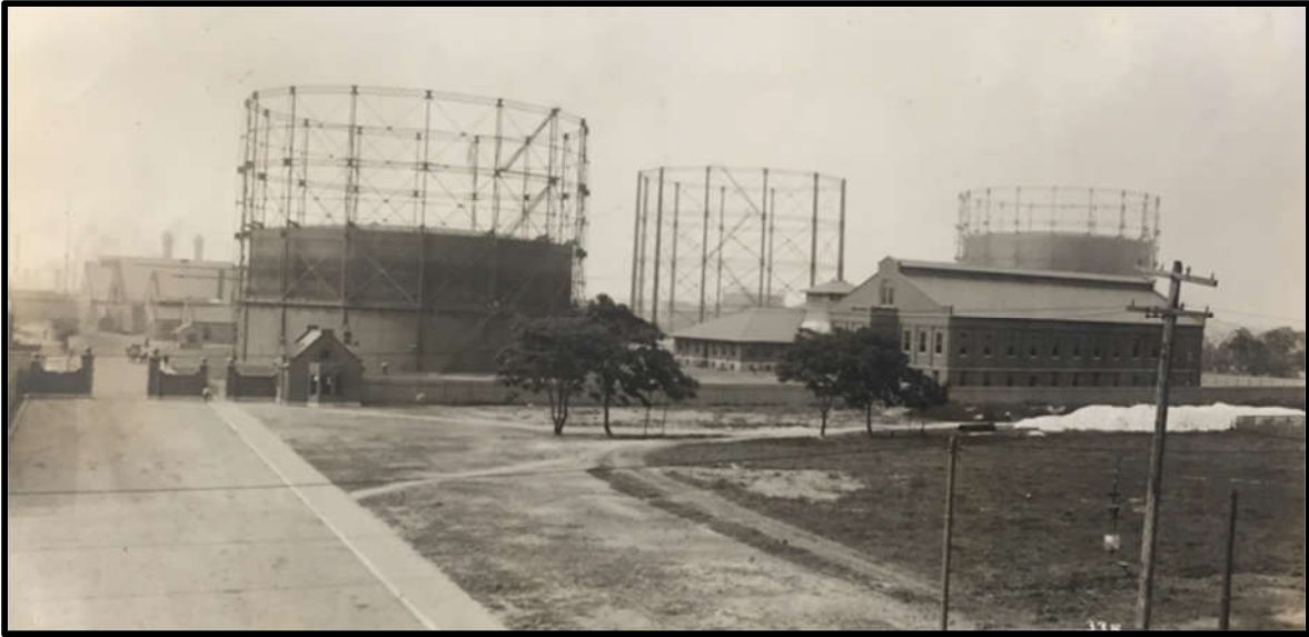
“Sta. A. Showing Relief Holder, Purifying House and end of Pusher, Valve, and Meter House, Auth. 51. Also entrance gates and gate house. Auth. 121. 1899–1900. Board Fence, Auth. 118, 1900.” Source: The PGW Photograph Collection, CAP.
