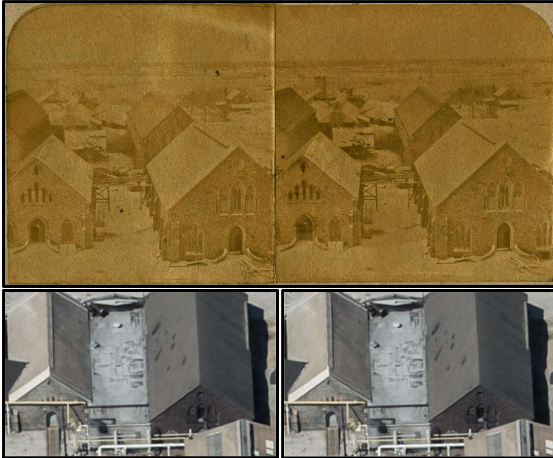
Figure 81. Top: Taken by Charles Massey Cresson, c. 1859–60, this view of the Point Breeze Gas Works showcases the northeast elevations of Resource No. 2: Purifying House (1859) on left and Resource No. 5a: Purifying House (1859) on right. Source: Library Company of Philadelphia. Figure 82. Bottom: Looking southwest at the northeast elevation of Resource No. 2: Purifying House (1859) on left and Resource No. 5a: Purifying House (1859) on right.
