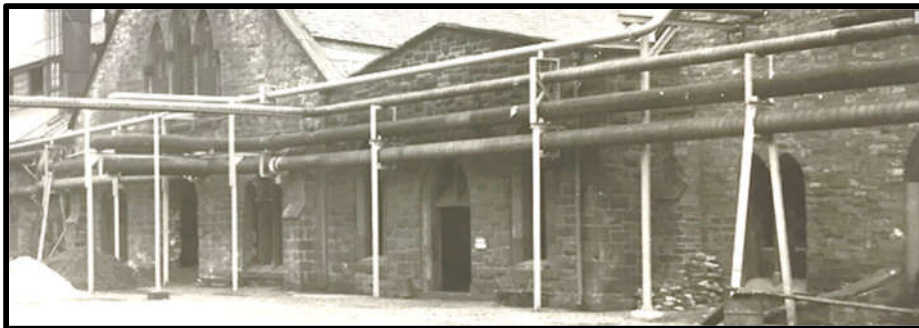
Figure 43. The primary (southwest) elevation of Resource No. 5b: Purifying House (1888–94). Source: The PGW Photograph Collection, CAP.
