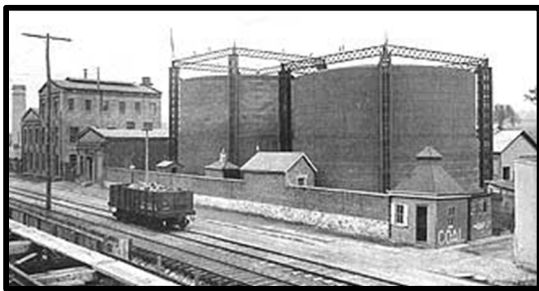
Reading Gas Light Company's Works at Canal and South Sixth Street, c. 1905. While some late nineteenth century buildings appear to be extant at the site, there are no buildings and/or structures that date to the foundational period of the company. Source:
