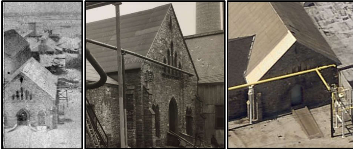
Figure 28. Left: The northeast elevation of Resource No. 2: Purifying House (1855) in a photograph taken c1859–60. Source: Library Company of Philadelphia. Figure 29. Center: The northeast elevation of Resource No. 2: Purifying House (1855), dated 1948. Source: The PGW Photograph Collection, CAP. Figure 30. Right: The northeast elevation of Resource No. 2: Purifying House (1855). Source: Atlas, City of Philadelphia, 2018.
