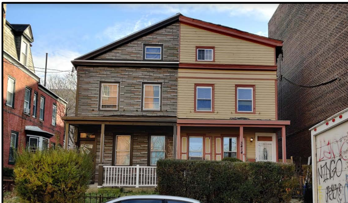
Figure 1 repeated. Source: Oscar Beisert, 2019.
