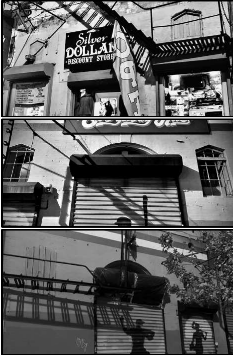
Top: Figure 15. A round-arch opening with flanking windows, showing the use of the low, arched top. Figure Center: 16. Another round-arch opening with flanking windows, showing the employment of the low, arched top, as well as the keystone in the round arch. Bottom: Figure 17. Another round-arch opening and its flanking windows. Source: Oscar Beisert, 2019.
