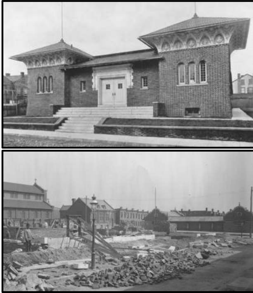
Civic-minded bathhouses by Hazelhurst & Huckel that were commissioned by the City of Philadelphia. Figure 48. Left: The 23 rd Ward Bathhouse, Hedges Street, Philadelphia, designed by Hazelhurst & Huckel in 1898 (demolished). Figure 49. Right: The 33 rd Ward Bathhouse, North Howard Street near Ontario, designed by Hazelhurst & Huckel in 1900 (demolished) can be seen in the background, a distinctive and fanciful public edifice structure defined by its small scale created through several building components. Source: DOR Archives, City Archives of Philadelphia.
