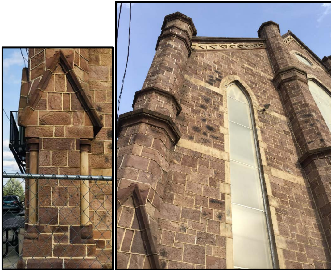
Figure 20. Left: A detail shot of the buttress at the base of the octagonal turret at the northwest corner of the building, showing its gable-front supported by colonettes. Figure 21. Right: The primary (west) elevation of the subject property, showing the northern most bay with a pointed arch window, a window hood, an octagonal tower and pilaster, and the Gothic-inspired cornice. Source: Oscar Beisert, 2019.
