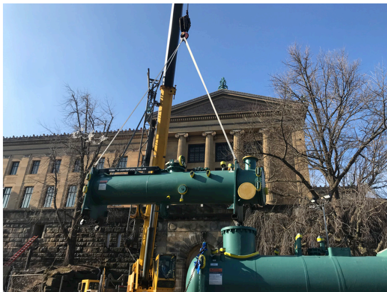
Workers outside the Philadelphia Museum of Art lift a new, high-efficiency chiller off the delivery truck.
