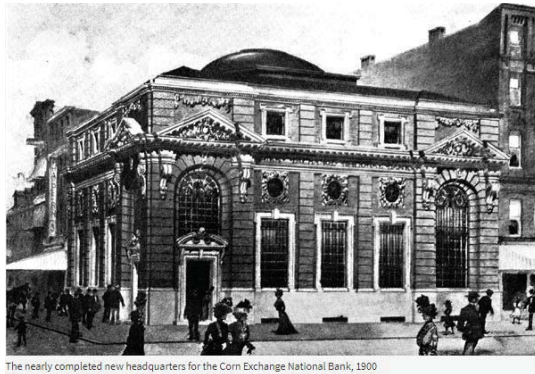
The nearly completed new headquarters for the Corn Exchange National Bank, 1900
