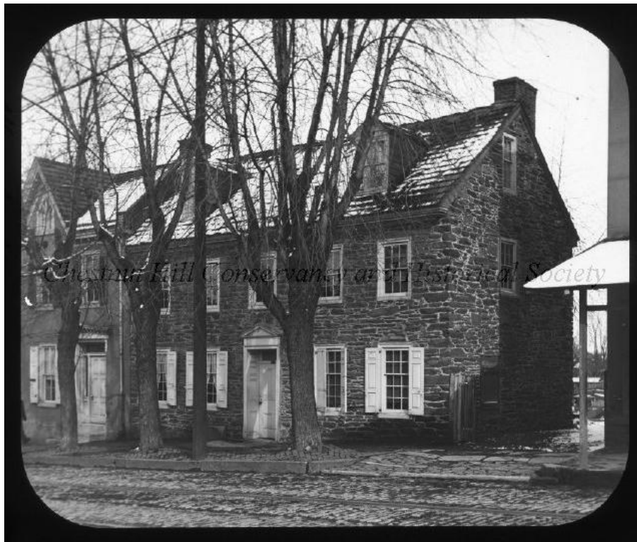
Figure 14. 7137 Germantown Avenue, demolished for the Sedgwick Theatre. (Chestnut Hill Conservancy)
