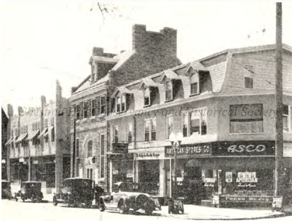
Figure 11. The west side of Germantown Ave., looking south at Mt. Airy Ave. the ASCO building is 7212-7216 Germantown Ave. The photo is undated, but the presence of the Tourison Building (left) places it after 1929. (Chestnut Hill Conservancy)
