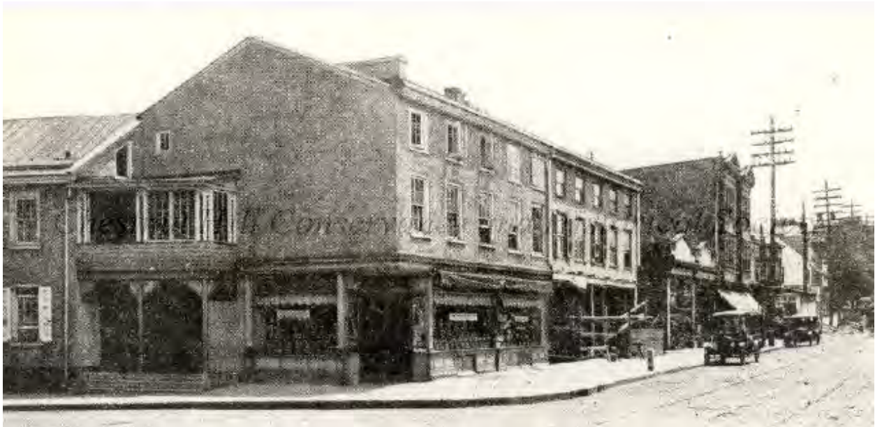
Figure 10. East side of Germantown Ave. looking south from the intersection of Mt. Airy Ave. The Shermer House (7169) is on the corner at the center, the Haas house at 7165 to its right, and then the three-story 7153-55. The photo is undated, but the presence of 7153-55 places it after 1915. (Chestnut Hill Conservancy)
