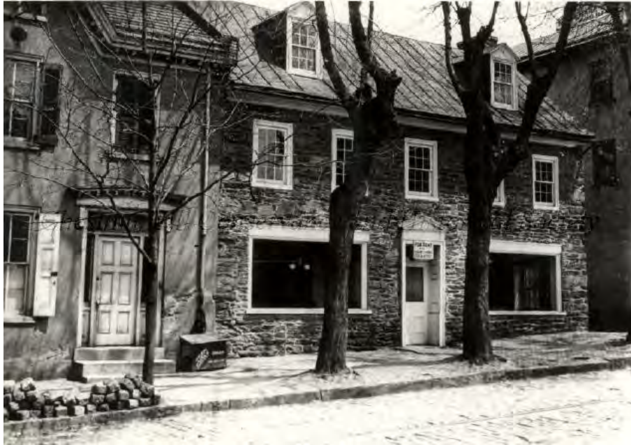
Figure 15. 7141 Germantown Avenue, demolished for the Sedgwick Theatre. (Chestnut Hill Conservancy)
