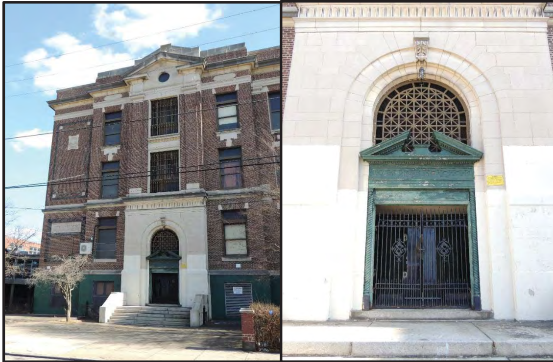
Figure 24. Left: The northeastern section of the northwest elevation of the 1914–16 Building. Figure 25. Right: a detail shot of the northeastern entrance within the primary (northwest) elevation. Source: Nicholas Covolus, 2018.
