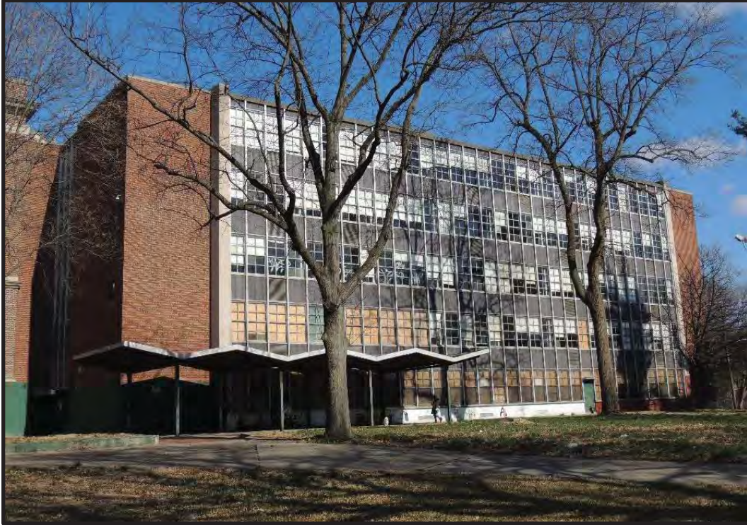
Figure 44. The southwest elevation of the 1959–60 Addition. Source: Nicholas Covolus, 2018.
