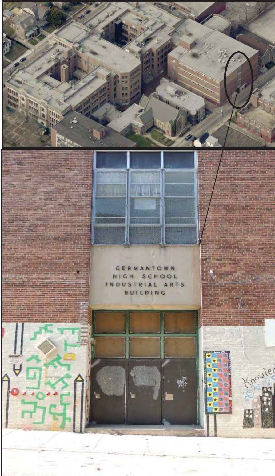
Figure 54. Top: Looking north at the subject property with the southeast elevation of the 1967–68 Addition circled to correspond with the photo displayed immediately above this caption. Figure 55. Bottom: Right: The southeast elevation of the 1967–68 Addition. Source: Nicholas Covolus, 2018
