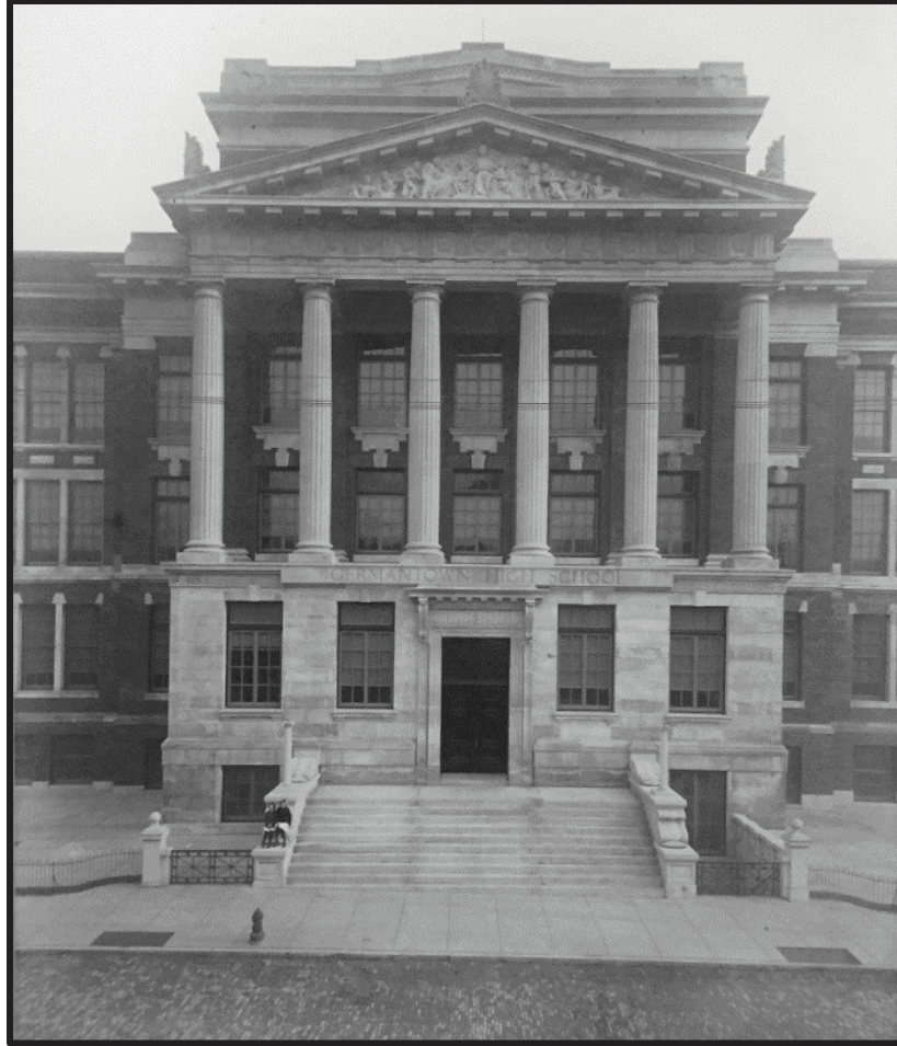
Figure 100. The northwest elevation of the 1914–16 Building of Germantown High School. Source: Historic Germantown.
