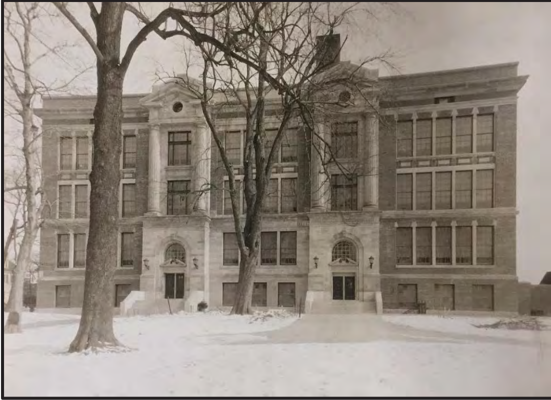
Figure 101. The southwest elevation of the 1914–16 Building of Germantown High School. Source: Photographs, Board of Education Records, CAP.
