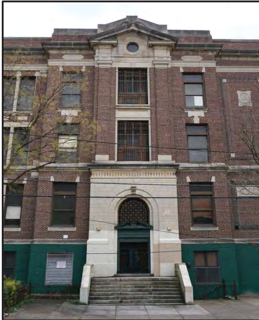
Figure 26. The southwest end of the primary (northwest) elevation, near the corner of the 1913–14 Building. Source: Oscar Beisert, 2018.
