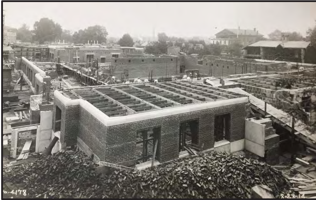
Figure 114. Looking northeast at the foundation of the 1914–16 Building of Germantown High School. Taken on 28 August 1914. Note: the stable of the Butler Mansion is being demolished on right in the background. Source: Photographs, Board of Education Records, CAP.
