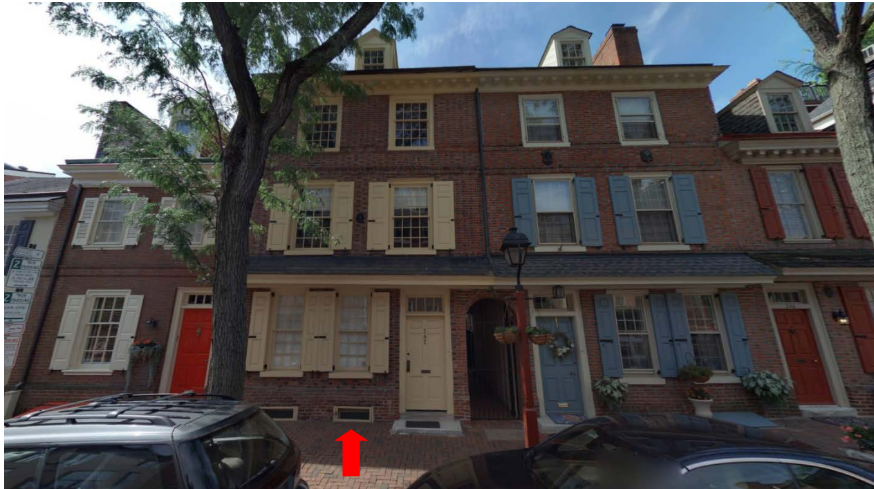
Figure 4: Front façade of 242 Delancey Street, 2019. Source: Cyclomedia.
