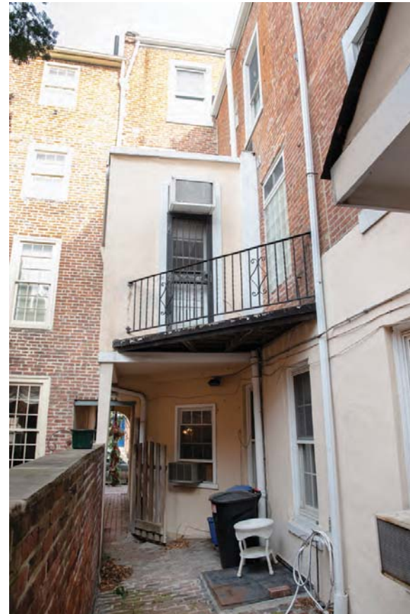
C4- INTERIOR COURTYARD PERSPECTIVE VIEW TOWARD NORTH (JAN 2020)
