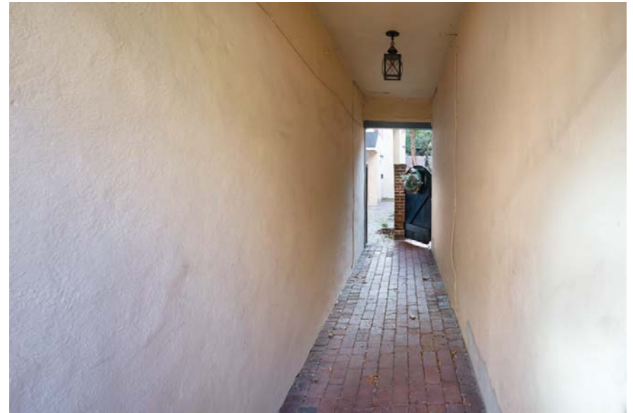
B4- VIEW OF INSIDE OF THE CORRIDOR (JAN 2020)
