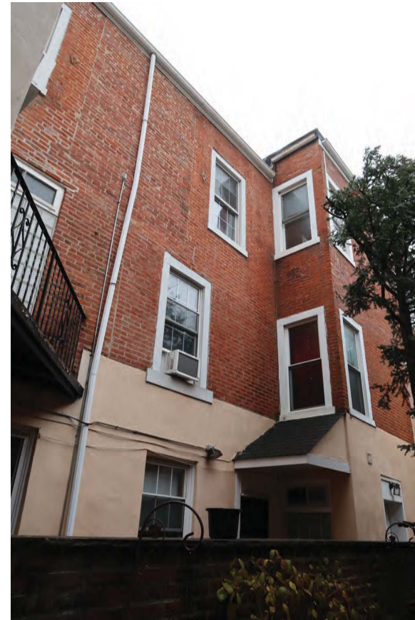
C2- WEST FACADE PERSPECTIVE TOWARD BACK OF THE HOUSE (JAN 2020)
