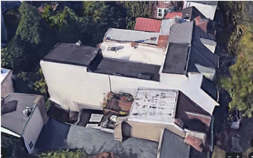
D1- AERIAL VIEW OF EAST FACADE OF THE BUILDING (GOOGLE IMAGE JAN 2020)
