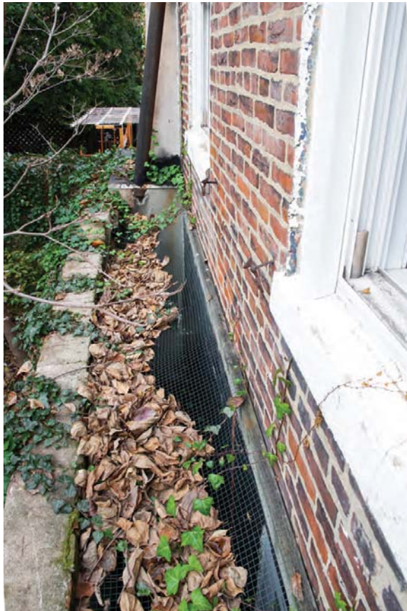
E3- BACK OF THE BUILDING VIEW FROM 2ND FL DOWN (JAN 2020)
