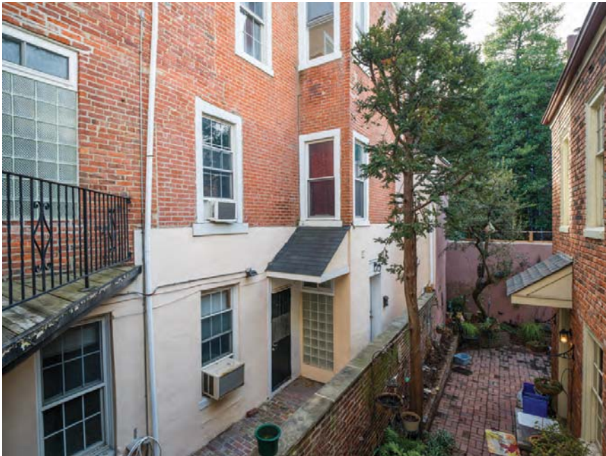
C7- INTERIOR COURTYARD PERSPECTIVE VIEW TOWARD SOUTH END (JAN 2020)
