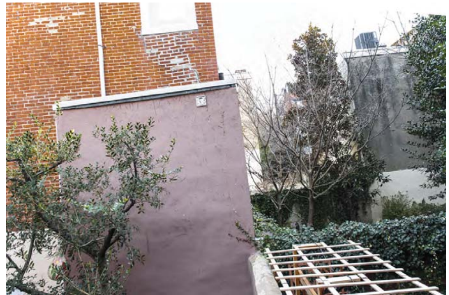
C10- INTERIOR COURTYARD OF THE BACK OF THE HOUSE FACING EAST AIR SHAFT BETWEEN HOUSE AND MASONRY WALL (JAN 2020)
