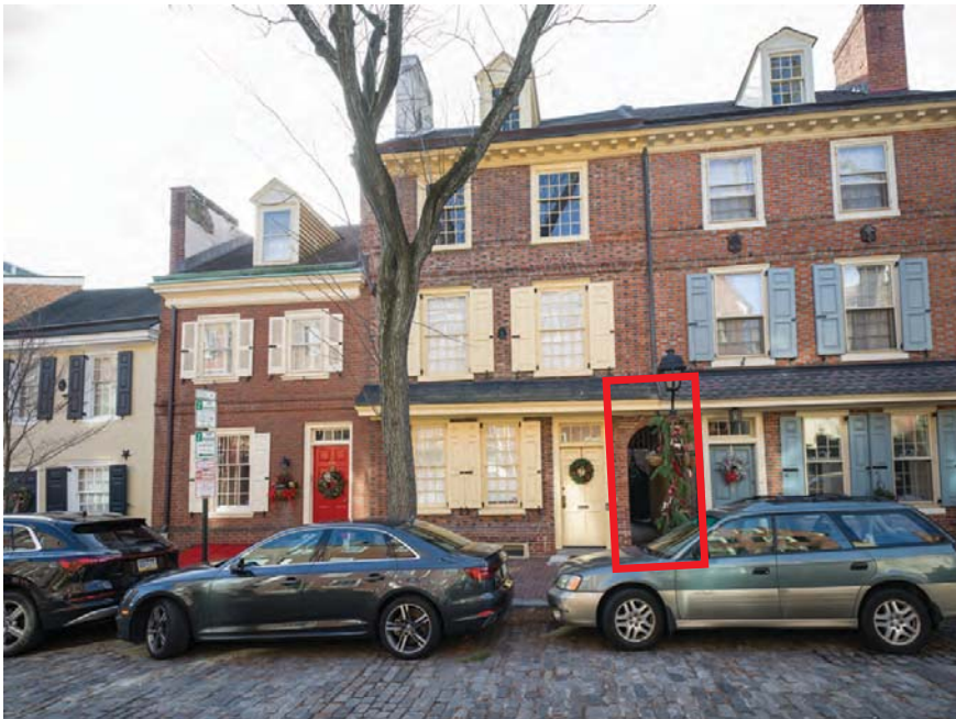
B1- NORTH FACADE OF THE BUILDING (JAN 2020)
