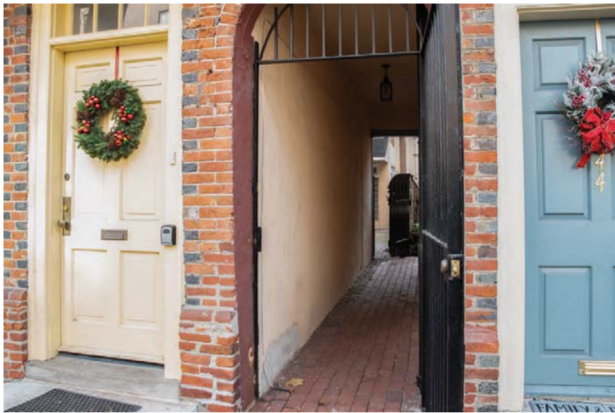
B3- CORRIDOR ENTRANCE FROM STREET VIEW (JAN 2020)
