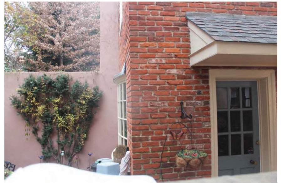
C12- EAST FACADE OF ADJACENT NEIGHBOR 244 DELANCEY ST. FACING WEST (DEC 2019)
