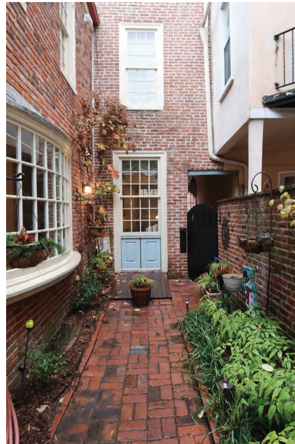
C14- INTERIOR COURTYARD OF ADJACENT NEIGHBOR 244 DELANCEY ST. FACING NORTH (DEC 2019)
