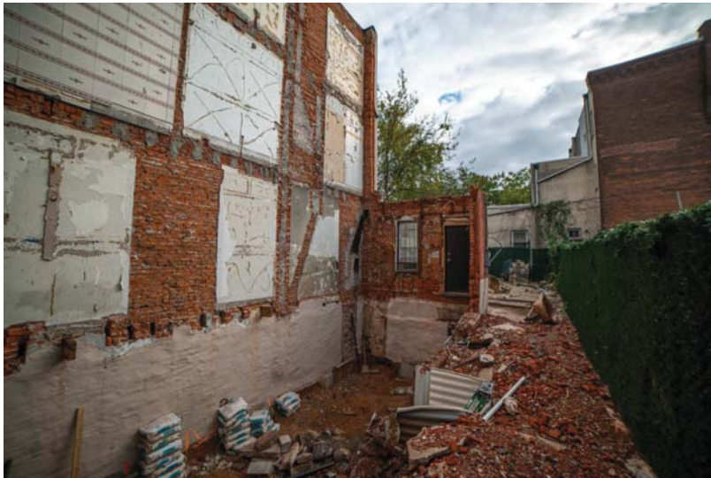
Side Rear that has been demolished by L&I
