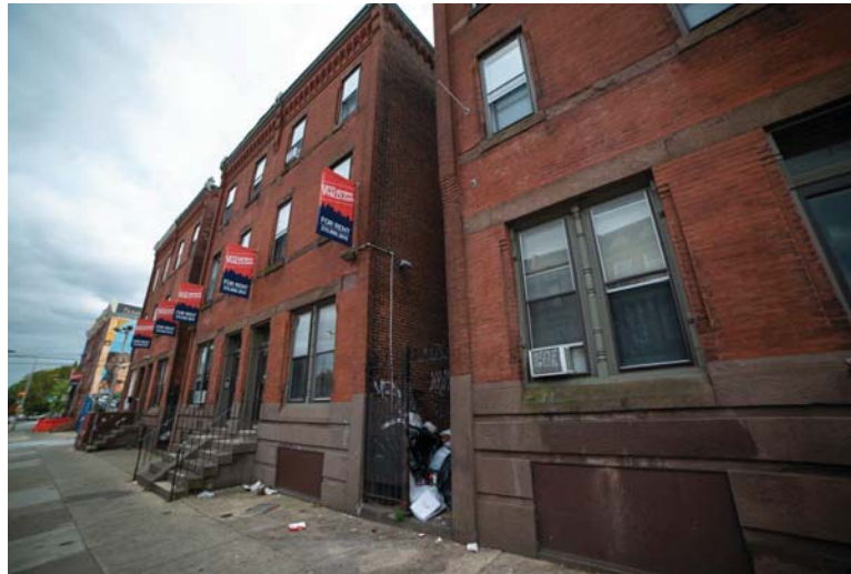
Side facade on a publi right-of-way on a angle
