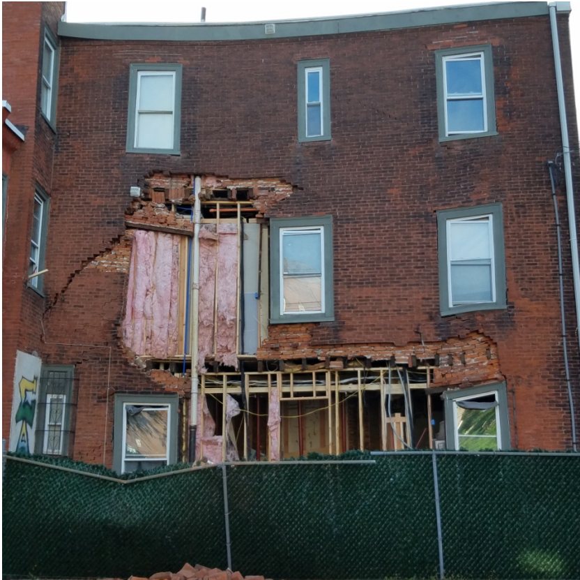
Figure 5: Partial collapse of the west wall of the rear ell, August 2019. Source: Philadelphia Historical Commission.
