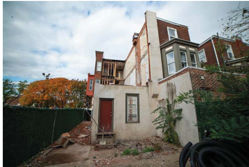
Rear of the building
