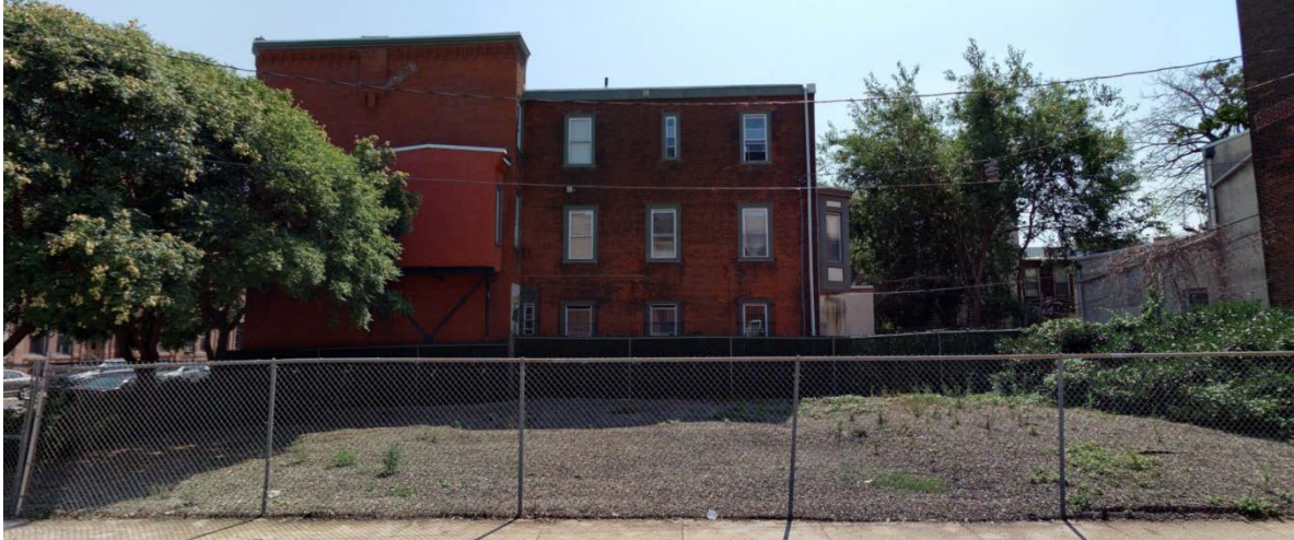
Figure 6: Side elevation of 1432 Diamond Street, showing the main block and rear ell prior to its demolition, 2019. Source: Cyclomedia.
