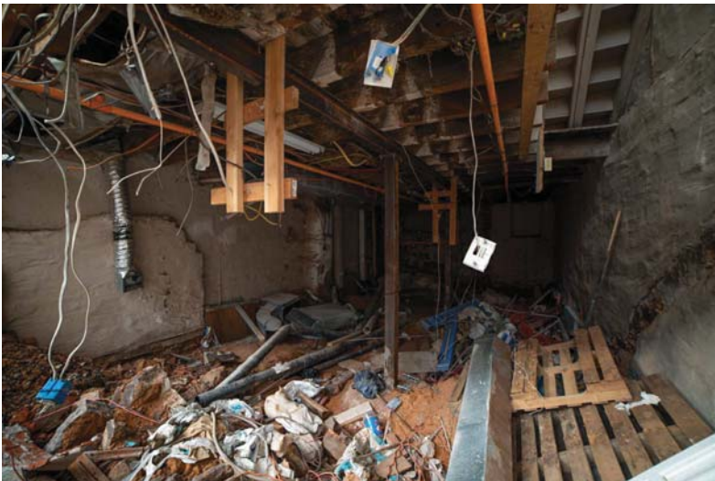
Inside the underpinning/basement portion
