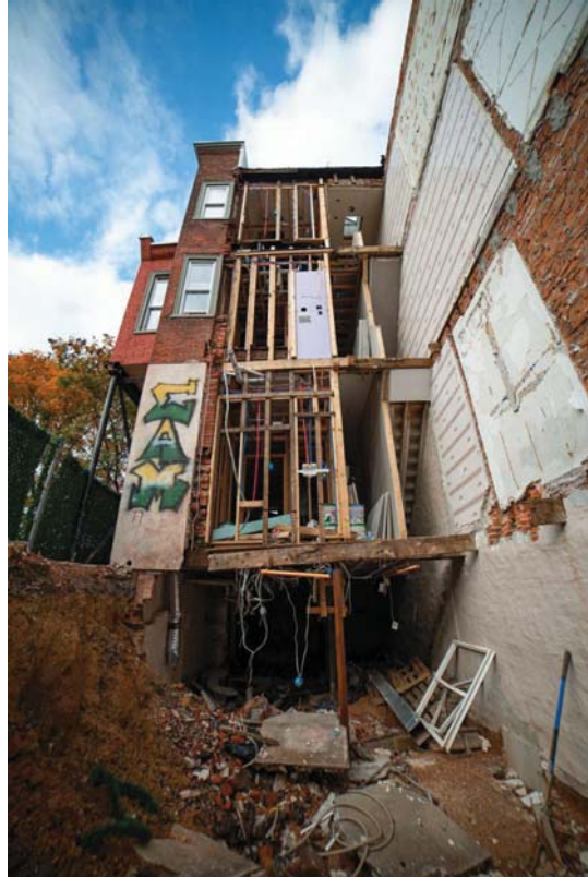
Rear portion of the 3story on a angle
