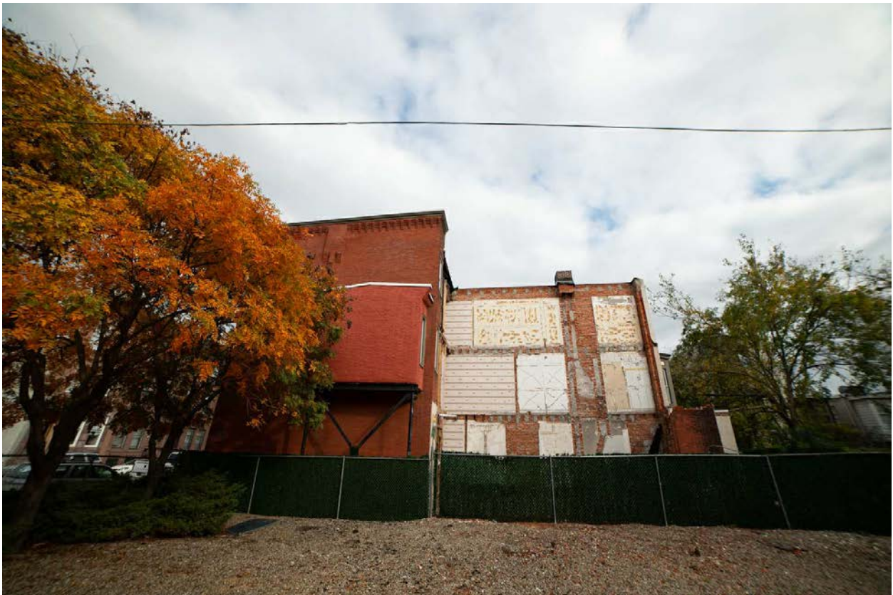
Figure 7: 1432 Diamond Street following the demolition of the rear ell, 2019. Source: Philadelphia Historical Commission.
