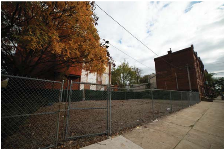
Side of building showing facing the rear on an angle on the public right-of-way
