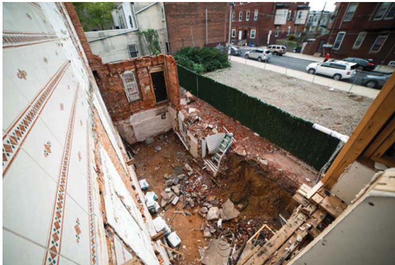
Portion of the rear that L&I demolished
