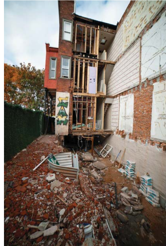
Full rear with underpinning
