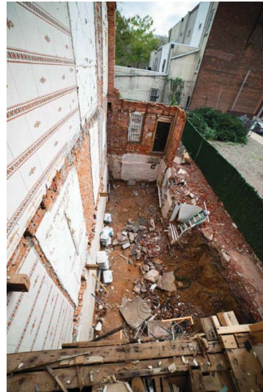
Rear portion of the underpinning
