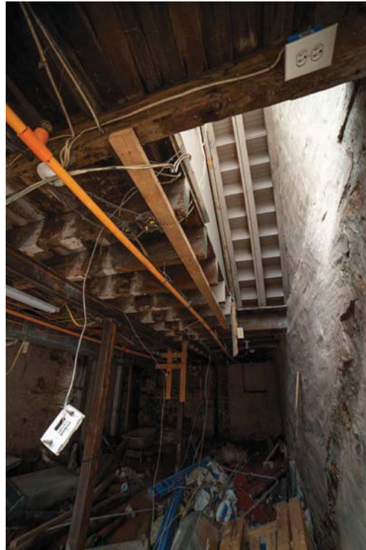
Inside the underpinning/basement portion
